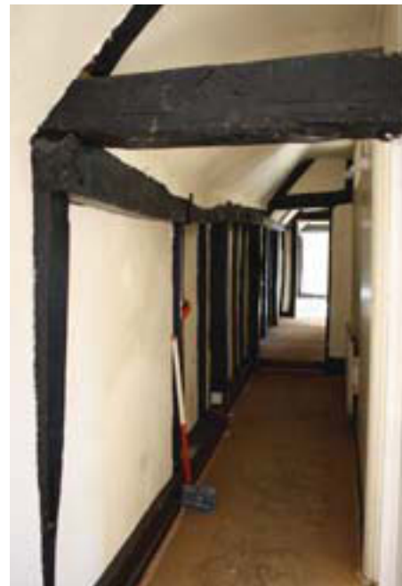
Plate 16. Interior, first floor corridor, looking west, Scales: 1m.
