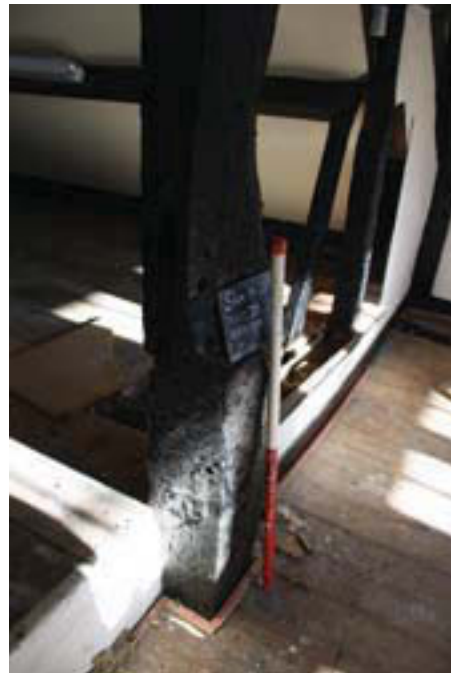
Plate 20. Interior, room 8 and 9 post detail, Scales: 1m.
