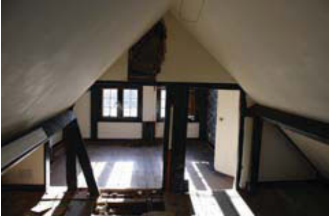
Plate 21. Interior, room 9, looking north, Scale: 1m.
