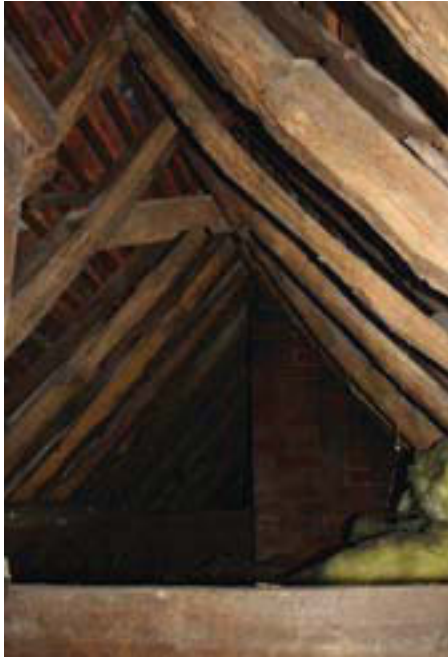
Plate 25. Interior, roof space, looking west.
