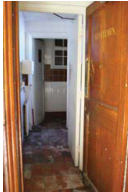
Plate 14. Interior, room 7, looking west, Scale: 1m.
