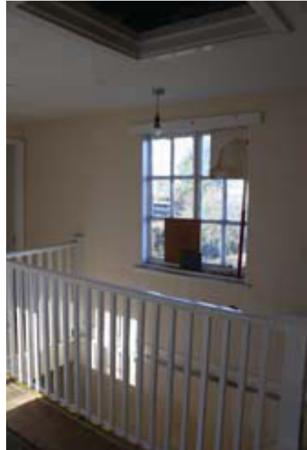
Plate 30. Interior, first floor, cottage room 3b, looking north west, Scale: 1m.
