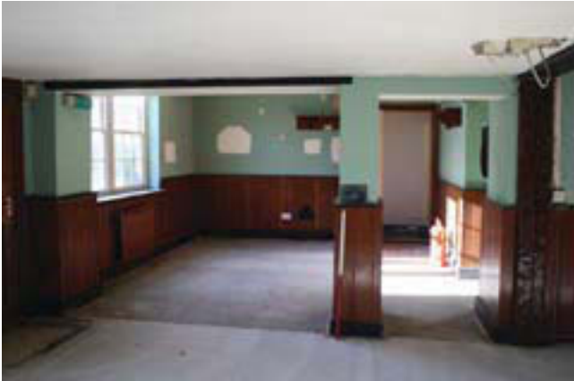
Plate 13. Interior, room 5, looking west, Scale: 1m.
