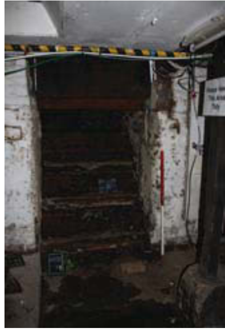
Plate 26. Interior, room 12, looking west, Scale: 1m.
