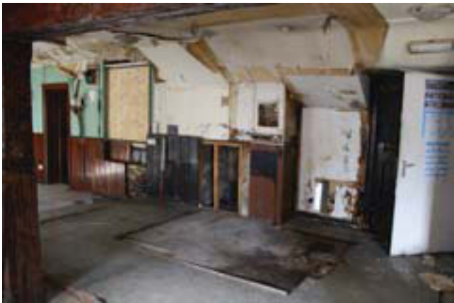
Plate 11. Interior, room 4, looking south, Scale: 1m.
