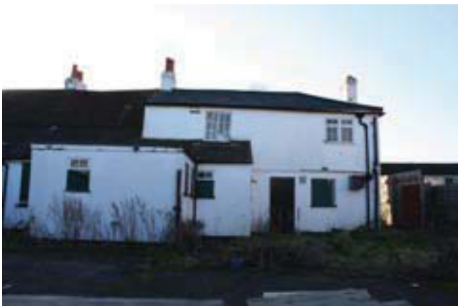
Plate 7. Exterior, rear elevation, looking south, Scale: 1m.
