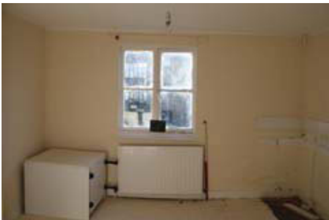
Plate 31. Interior, first floor, cottage room 4b, looking north, Scale: 1m.
