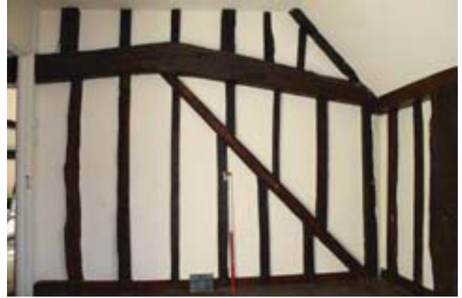
Plate 22. Interior, room 10 wall detail, Scale: 1m
