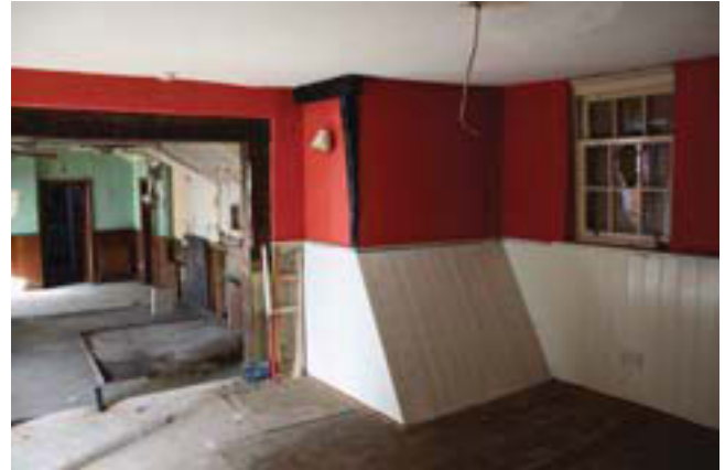
Plate 10. Interior, room 2 looking north west, Scale: 1m.
