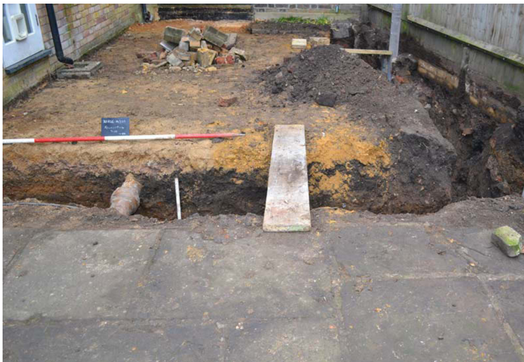
Plate 2. New footing, looking west, Scales: 2m and 1m.
