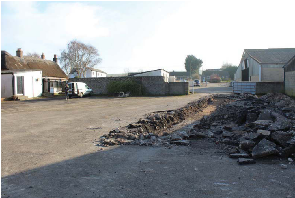
Plate 7. Trench 3, looking south east,
