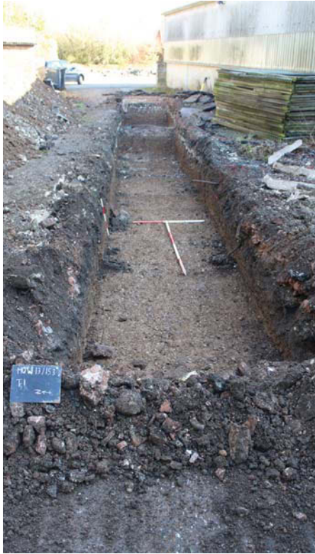
Plate 1. Trench 1, looking east, Scales: horizontal 2m and 1m, vertical 0.5m.
