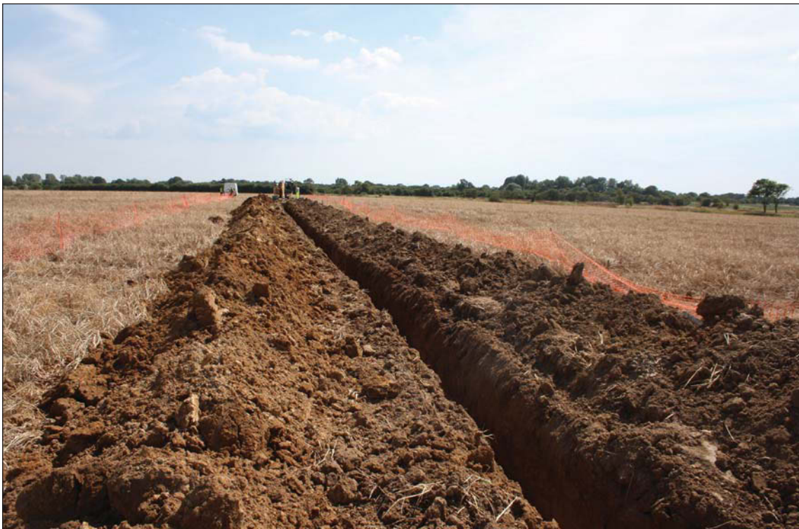
Plate 2. Cable Trench 1, looking north.
