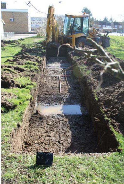
Plate 2. Trench 2, looking south-east, Scales: horizontal 2m and 1m, vertical 0.5m.
