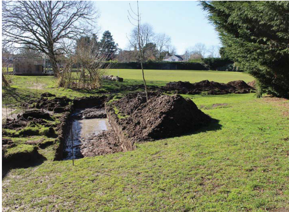
Plate 1. Location of trenches, looking south-west.
