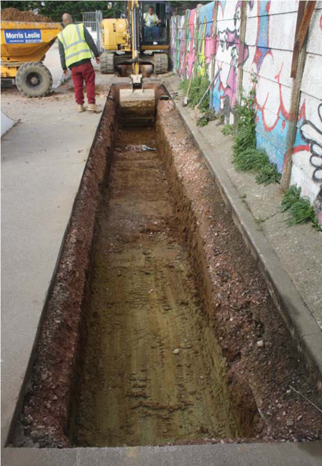
Plate 5. Boundary trench, Area A, looking NW.
