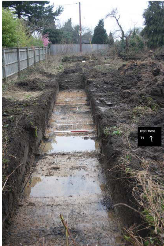
Plate 1. Trench 1, looking north, Scale: 1m.
