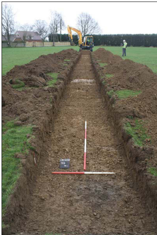
Plate 3. Trench 6, looking east. Scales: horizontal 2m and 1m, vertical 0.3m.
