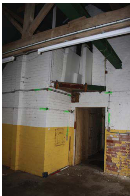
Plate 14. View to raised walkway above room 8, looking west, Scales: 2 x 1m.
