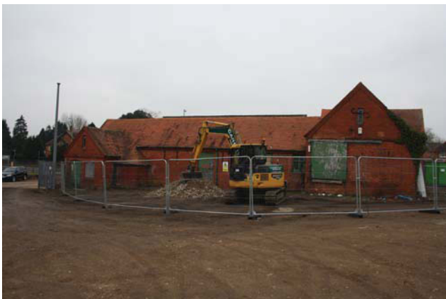
Plate 3. SE elevation, looking west.
