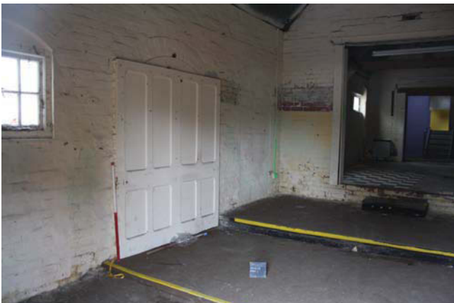
Plate 7. Blocked doors in room 1, looking north, Scales: 2 x 1m.
