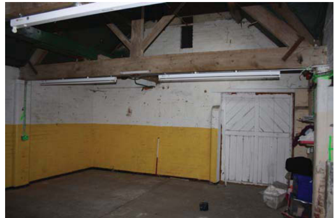
Plate 12. Door and blocked window within room 6, looking east, Scales: 2 x 1m.
