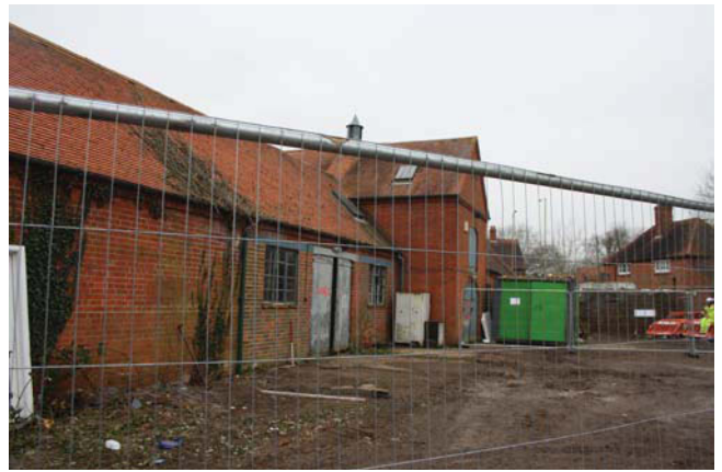
Plate 4. NE elevation, looking west, Scales: 2 x 1m.
