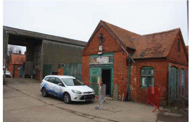
Plate 2. SW elevation, looking north, Scales: 2 x 1m.
