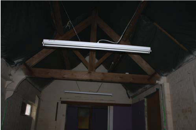
Plate 9. Roof truss within room 3, looking northeast.
