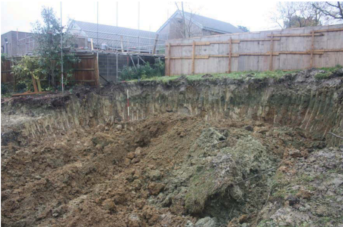
Plate 2. Garage terrace reduction, looking east, Scales: 2m and 1m.
