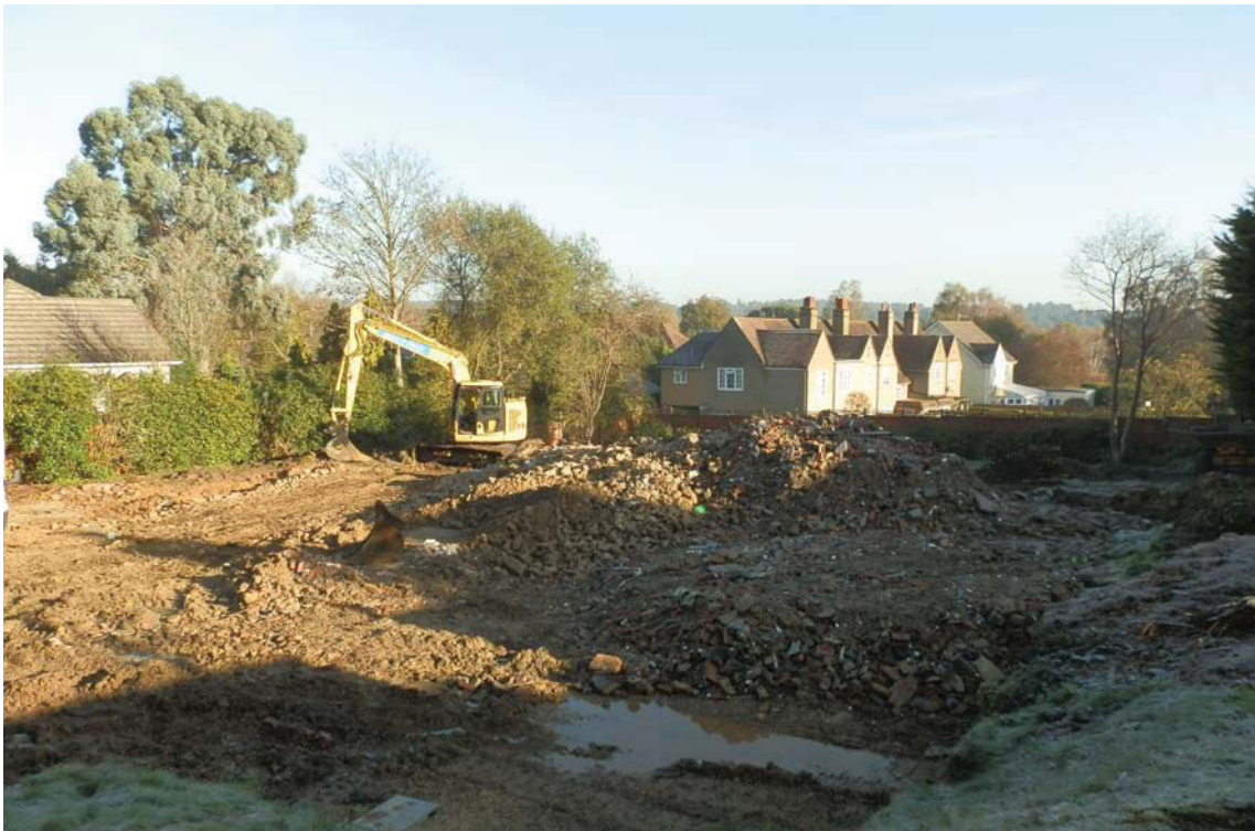
Plate 1. General view of the site, looking north
