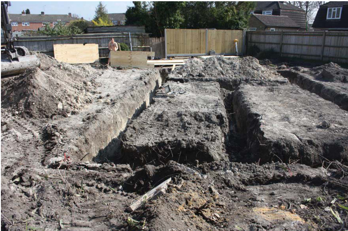
Plate 1. Extent of footings, looking south east.
