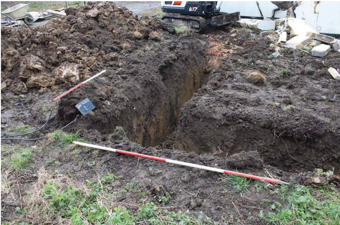
Plate 1. New footing trench, looking north east, Scales: 2m and 1m.
