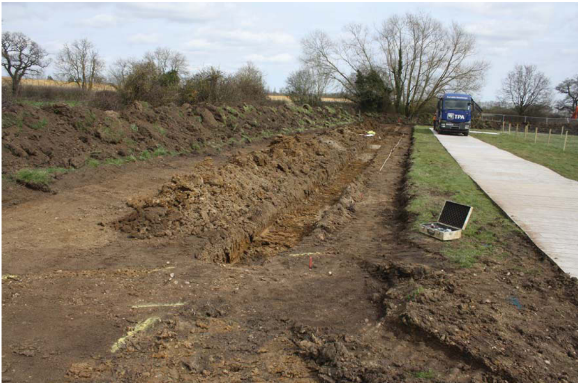
Plate 1. Pipe trench, looking east.
