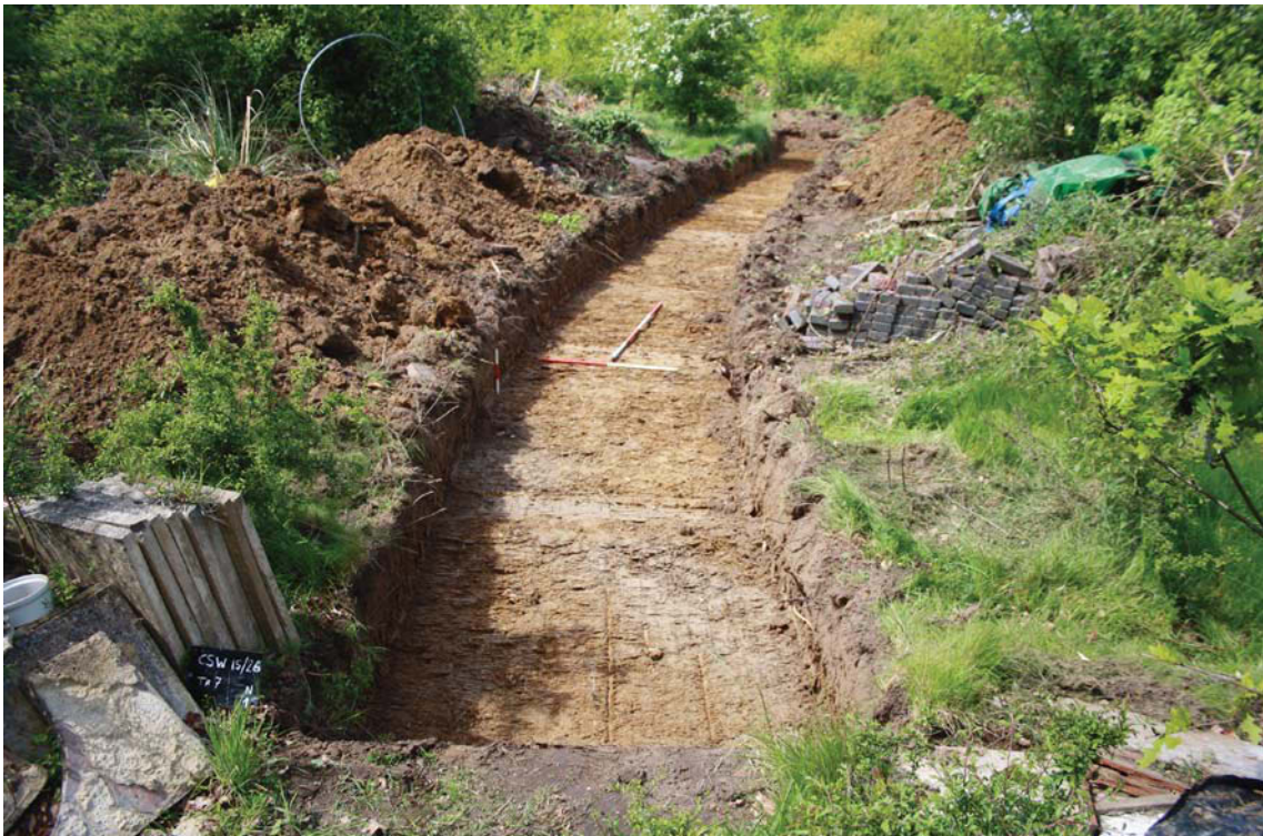
Plate 1. Trench 7, looking north west, Scales: horizontal 2m and 1m, vertical 0.3m.
