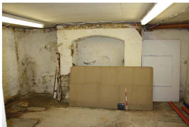
Plate 6. Room 43, view to fireplace base, looking southwest. Scale 0.5m.
