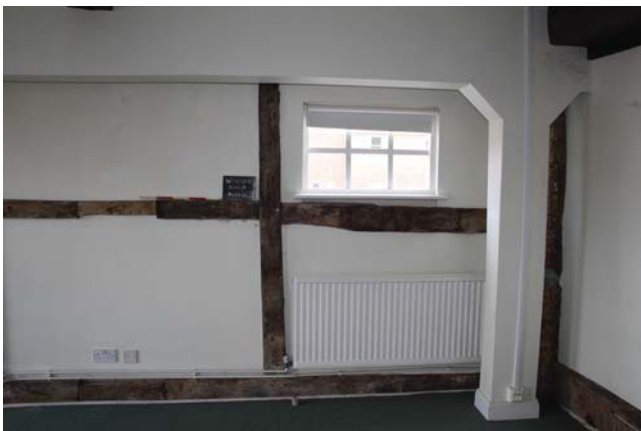
Plate 27. Room 29, timber detail, looking southeast. Scale 0.5m.
