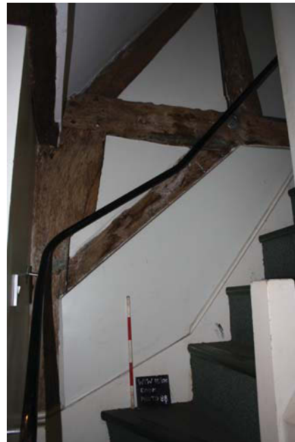
Plate 28. Room 25, detail of timber framing, looking west. Scale 0.5m.
