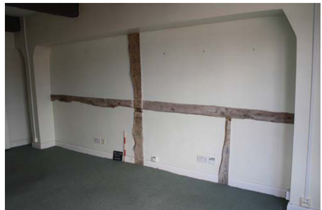
Plate 20. Room 26, timber framing detail, looking southwest. Scale 0.5m.
