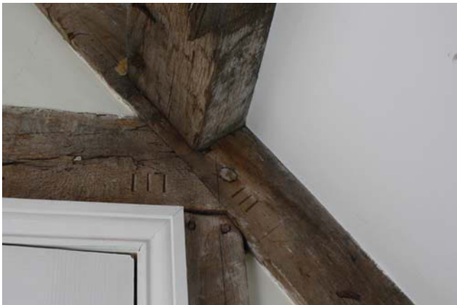
Plate 43. Room 40, detail of carpenter's mark (III), looking northwest.
