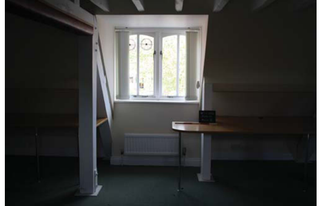
Plate 38. Room 37, To dormer window showing cut purlin, looking northeast. Scale 0.5m.
