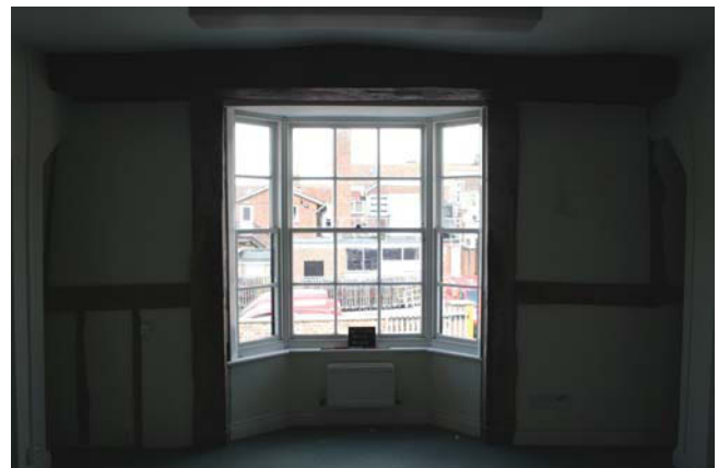
Plate 24. Room 28, bay window and timber framing detail, looking north. Scale 0.5m.
