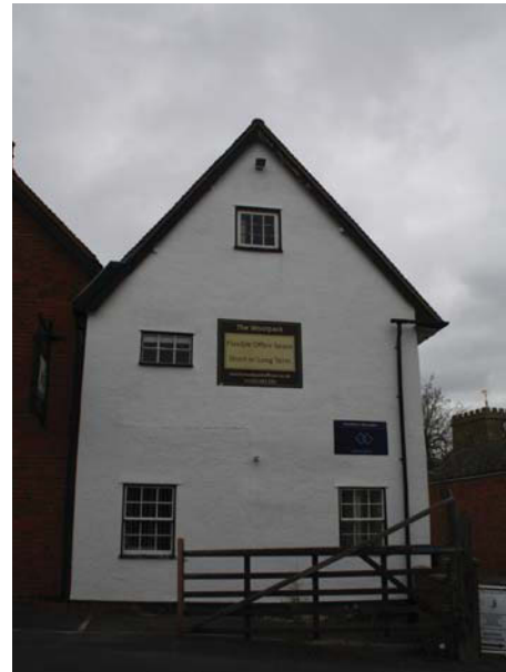
Plate 2. Exterior, gable, east facing.
