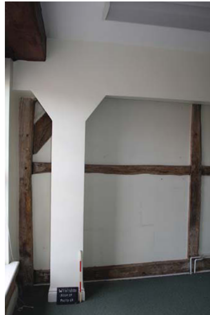
Plate 26. Room 29, timber detail, looking southeast. Scale 0.5m.
