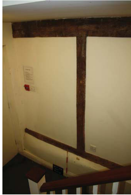
Plate 14. Room 7, timber framing, looking northwest. Scale 0.5m.
