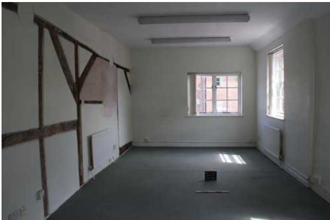
Plate 31. Room 30, along room to windows, looking southeast. Scale 0.5m.
