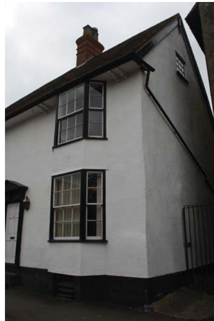
Plate 4. Exterior, window detail on frontage (north western corner), looking south east.
