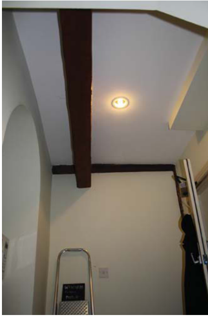
Plate 13. Room 6, timber detail in ceiling, looking east.
