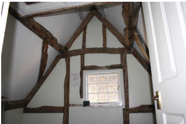
Plate 39. Room 39, gable end, looking northwest. Scale 0.5m.
