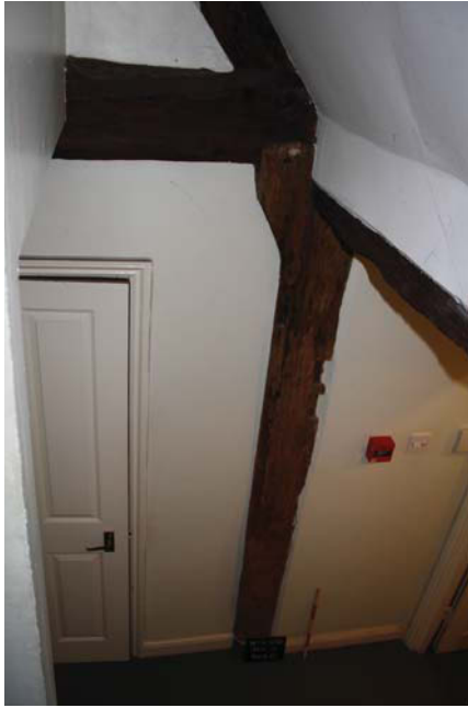
Plate 29. Room 25, timber framing detail, looking east. Scale 0.5m.
