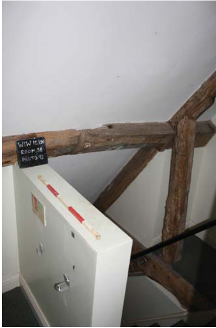
Plate 41. Room 38, detail of purlin jointing, looking west. Scale 0.5m.
