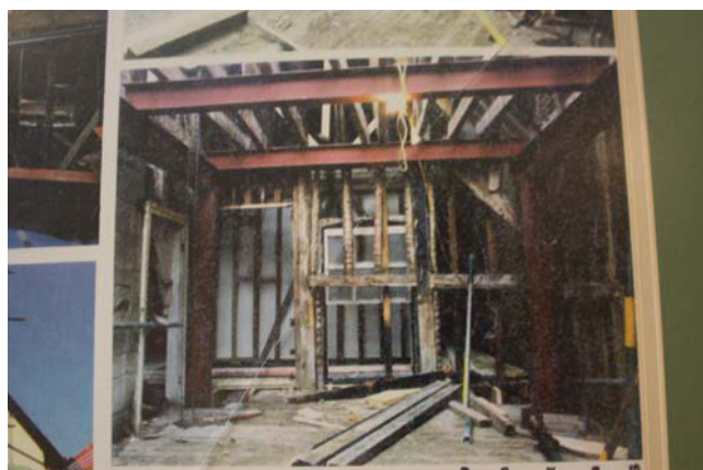
Plate 8. Room 1, looking north (1990 renovation).
