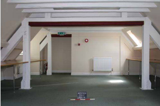
Plate 37. Room 37, General view showing roof structure, looking south. Scale 0.5m.
