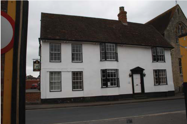
Plate 1. Exterior, front elevation (Church Street), looking south.
