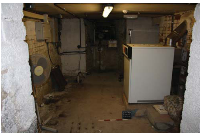
Plate 7. Room 44, view to beer slide, looking northeast. Scale 0.5m.
