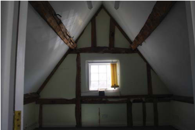
Plate 45. Room 41, gable end, looking southeast. Scale 0.5m.
