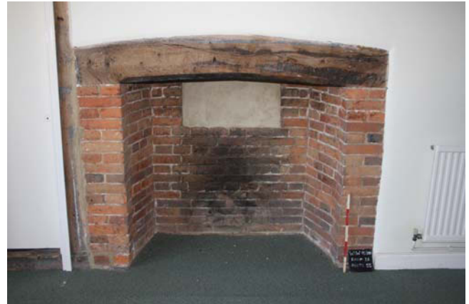
Plate 22. Room 26, fireplace detail, looking east. Scale 0.5m.
