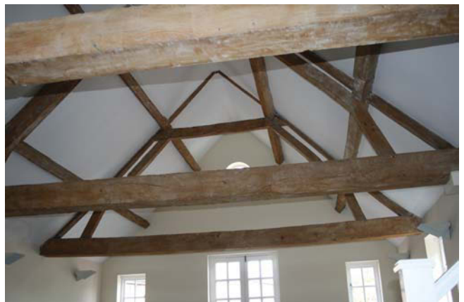
Plate 36. Room 36, roof trusses, looking east.
