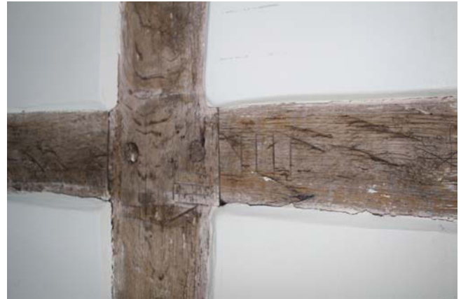
Plate 34. Room 30, carpenter's mark 'VIII', looking northeast.
