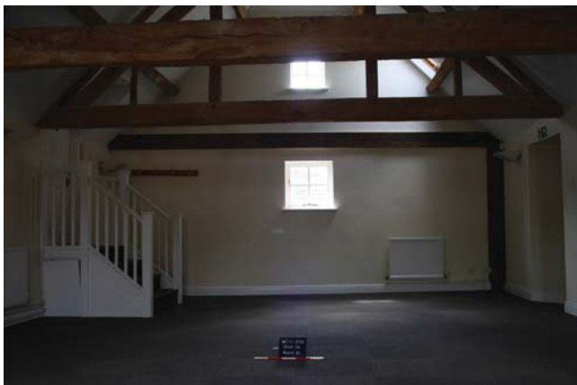
Plate 35. Room 36, view to windows showing trusses, looking west. Scale 0.5m.
