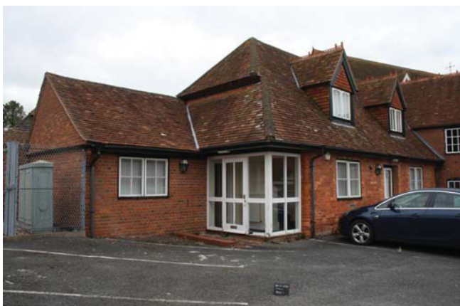
Plate 5. Exterior, rear extension, looking north west.
