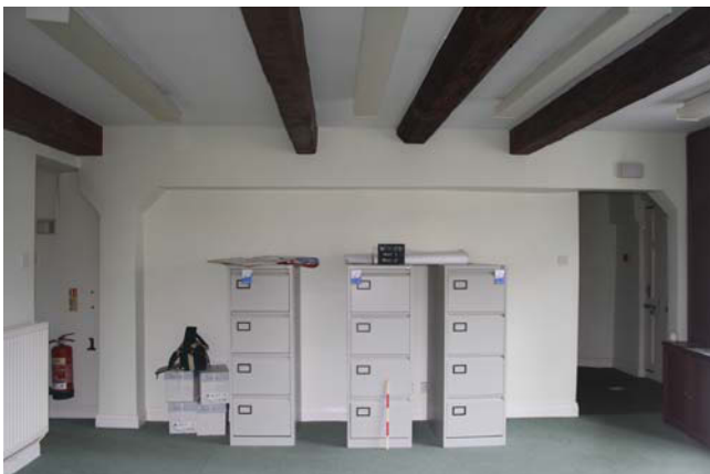
Plate 11. Room 3, to west wall showing beams, looking west. Scale 0.5m.
