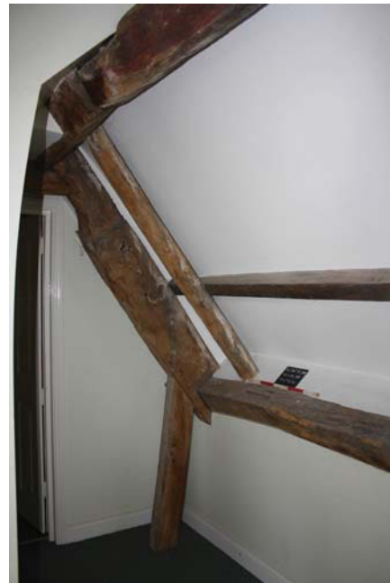
Plate 40. Room 38, detail of roof structure, looking northwest. Scale 0.5m.
