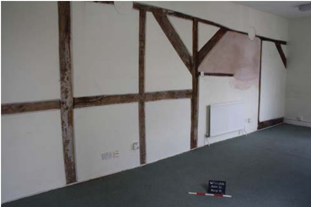
Plate 33. Room 30, timber framing detail, looking northeast. Scale 0.5m.
