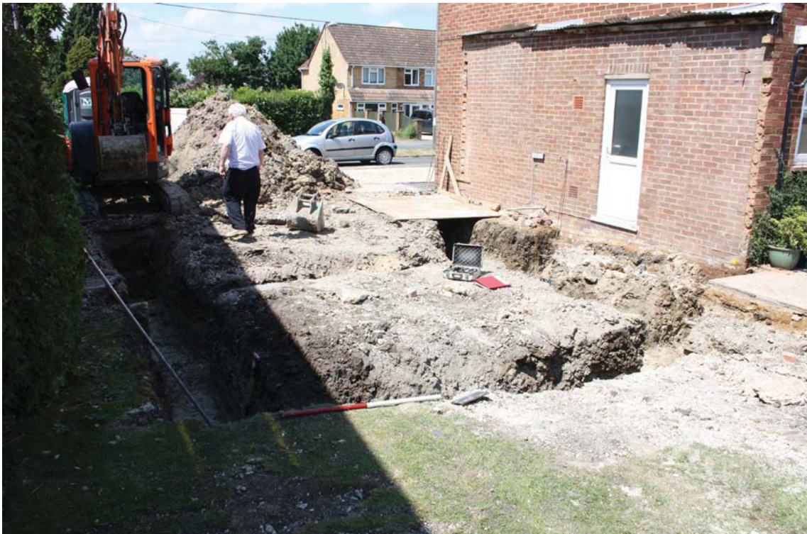
Plate 1. View of new footings, looking north, Scale: 1m.
