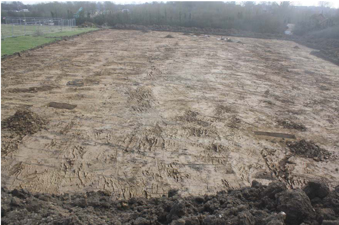
Plate 1. Stripped area, looking south.
