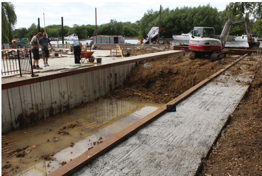
Plate 1. Excavating the wet dock, looking west
