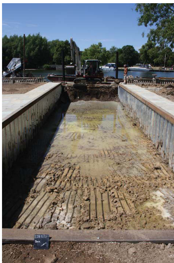
Plate 2. Excavated wet dock, looking northwest.
