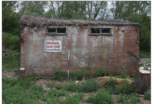
Plate 4. East facing elevation of structure A. Scales: 2m and 1m.
