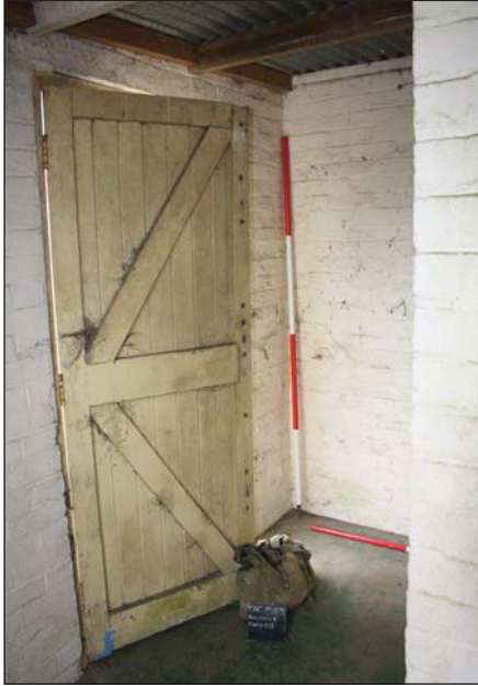
Plate 13. Door in ladies toilet looking north-east. Scales: 2m and 1m.
