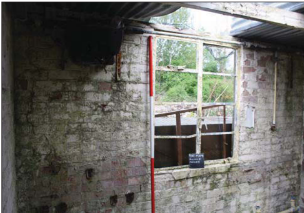
Plate 15. Crittall style window in mens toilet, looking north-west. Scale: 2m.
