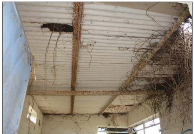
Plate 8. Roof detail within structure A, looking south.
