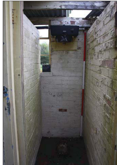
Plate 16. Mens toilet, looking east. Scale: 2m.
