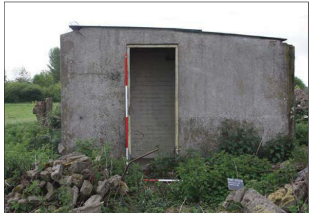
Plate 12. North facing elevation of structure B. Scale: 2m and 1m.
