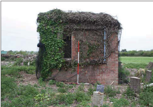
Plate 3. South facing elevation of structure A. Scales: 2m and 1m.
