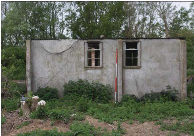
Plate 11. East facing elevation of structure B. Scale: 2m.
