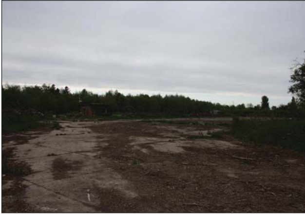
Plate 1. View to structures A and B, looking south-east
