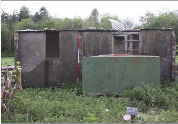
Plate 9. West facing elevation of structure B. Scales: 2m and 1m.
