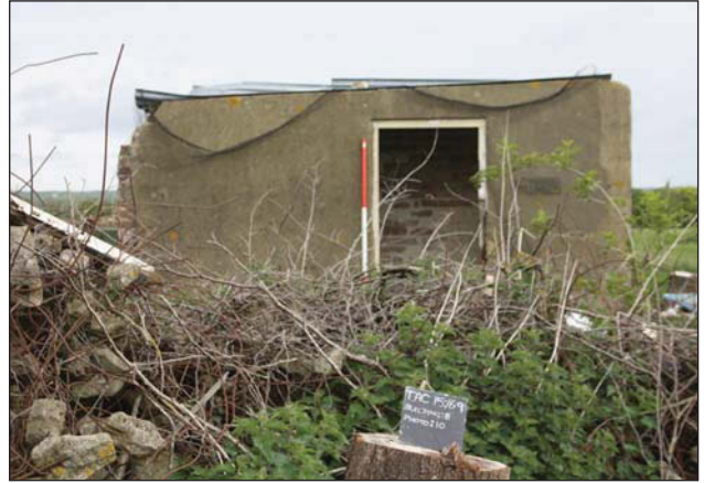
Plate 10. South facing elevation of structure B. Scale: 2m.
