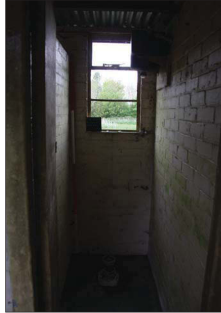
Plate 14. Ladies toilet, looking east. Scale: 2m.
