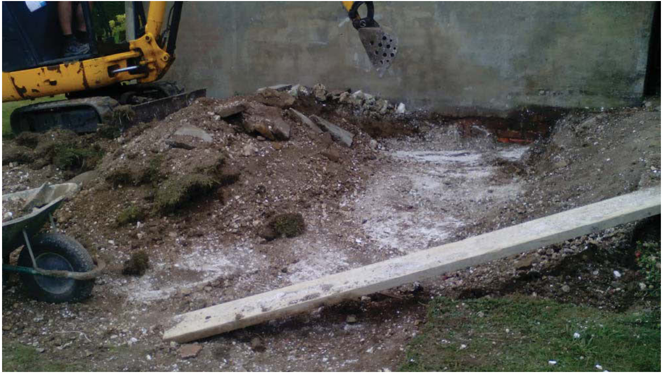
Plate 1: General view of site stripping, looking west
