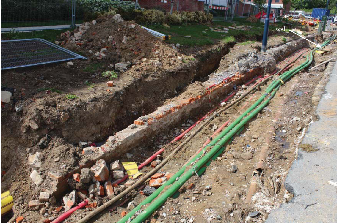
Plate 7. Area 4 pipe trench, looking north west, Scales: 2m and 0.5m.
