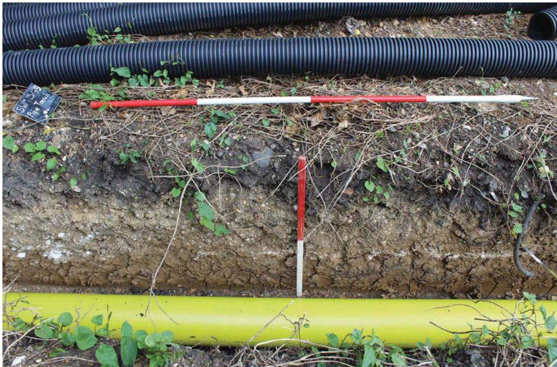
Plate 6. Area 3 pipe trench, looking east, Scales: 2m and 1m.
