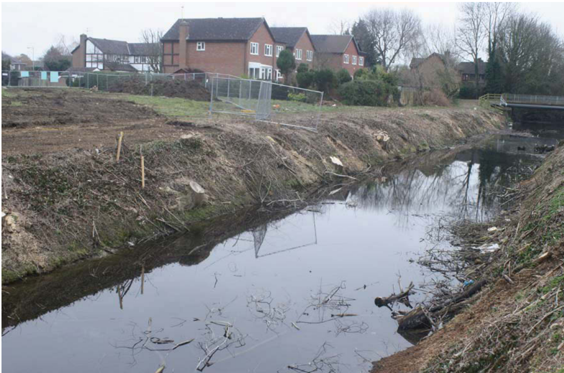
Plate 1. Bridging point, looking north west.
