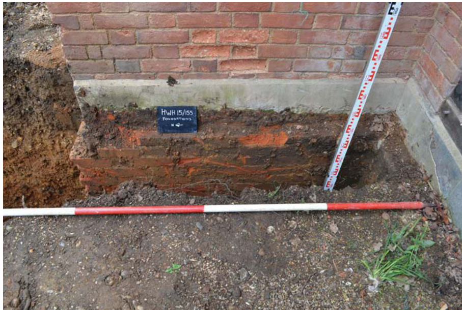
Plate 1. Foundation of house wall A, looking east, Scale: 2m.
