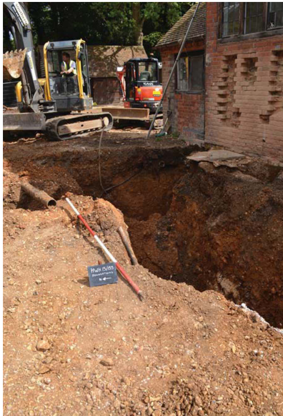
Plate 4. Trench D, looking south east, Scale: 2m.
