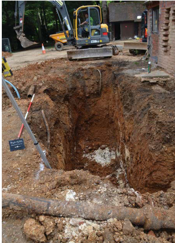
Plate 3. Trench C looking east, Scale: 2m.
