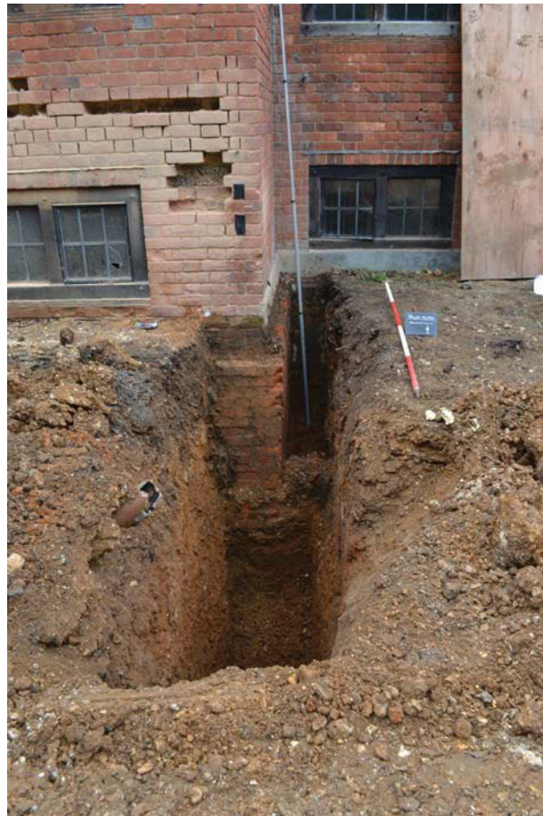
Plate 2. Trenches A and B, looking south, Scale: 2m.
