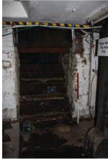
Plate 26. Interior, room 12, looking west, Scale: 1m.
