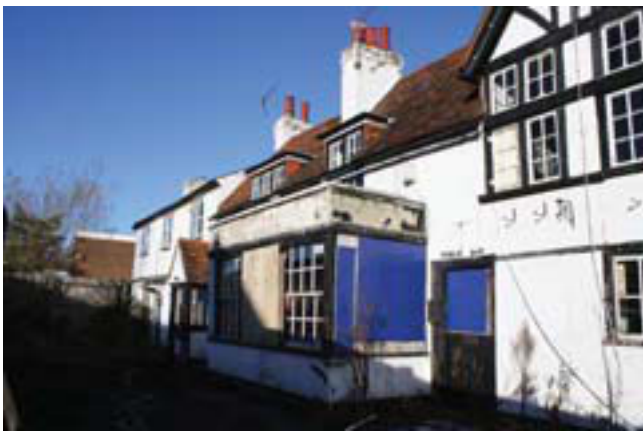
Plate 3. Exterior, front elevation, looking north west, Scale: 1m.
