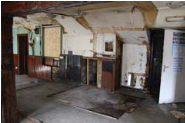
Plate 11. Interior, room 4, looking south, Scale: 1m.
