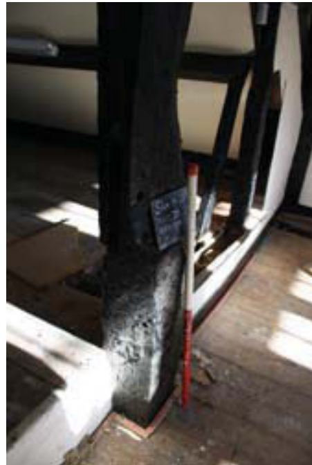
Plate 20. Interior, room 8 and 9 post detail, Scales: 1m.
