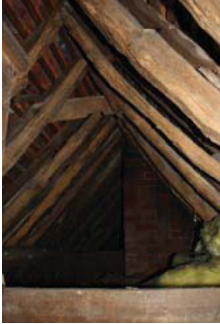
Plate 25. Interior, roof space, looking west.
