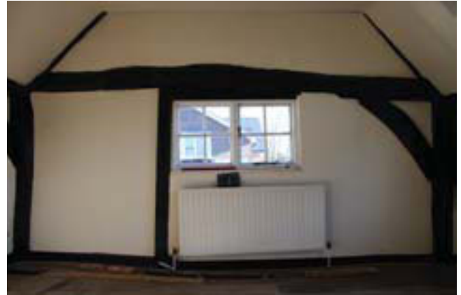
Plate 18. Interior, room 8, looking north, Scale: 1m
