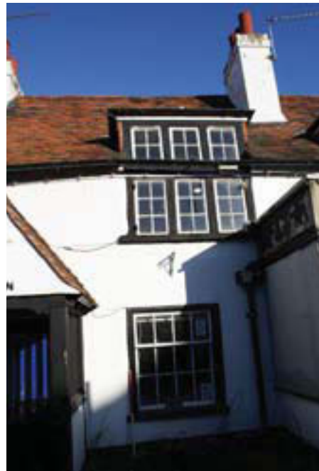
Plate 4. Exterior, frontage windows detail, looking north, Scales: 1m.
