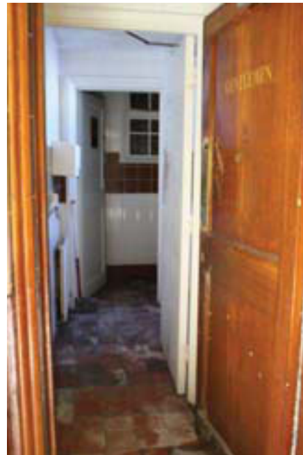
Plate 14. Interior, room 7, looking west, Scale: 1m.
