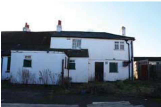
Plate 7. Exterior, rear elevation, looking south, Scale: 1m.
