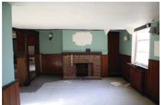
Plate 12. Interior, room 5 fireplace, looking east, Scales: 1m.
