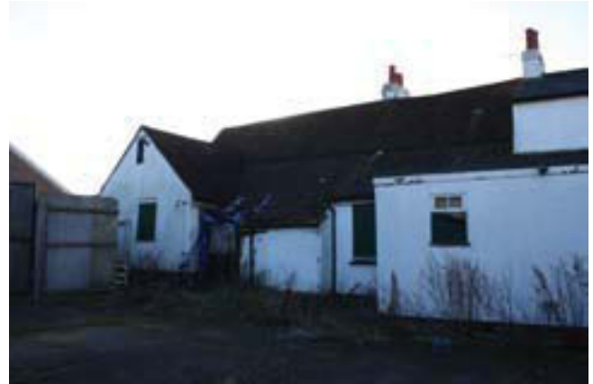
Plate 6. Exterior, rear elevation, looking north east, Scale: 1m
