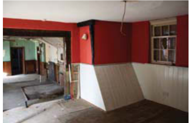
Plate 10. Interior, room 2 looking north west, Scale: 1m.
