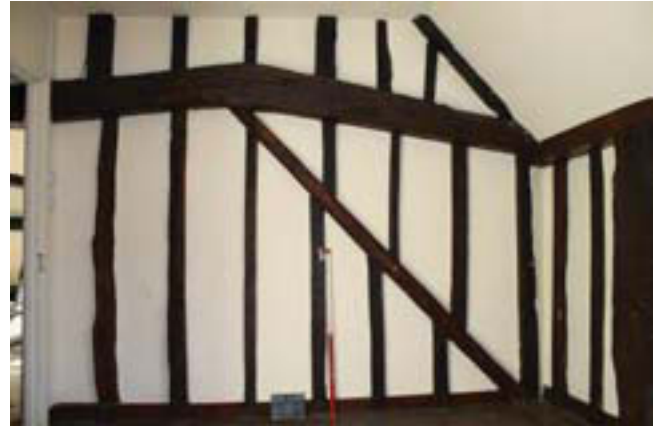
Plate 22. Interior, room 10 wall detail, Scale: 1m
