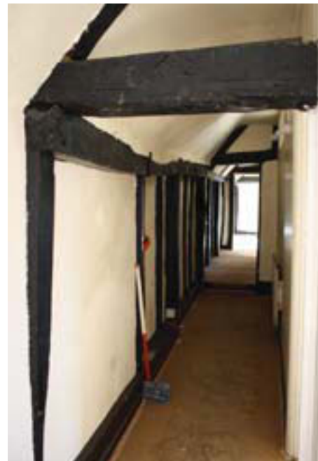
Plate 16. Interior, first floor corridor, looking west, Scales: 1m.
