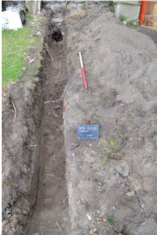
Plate 1. Trench 1, looking east, Scales: horizontal 1m, vertical 0.5m.
