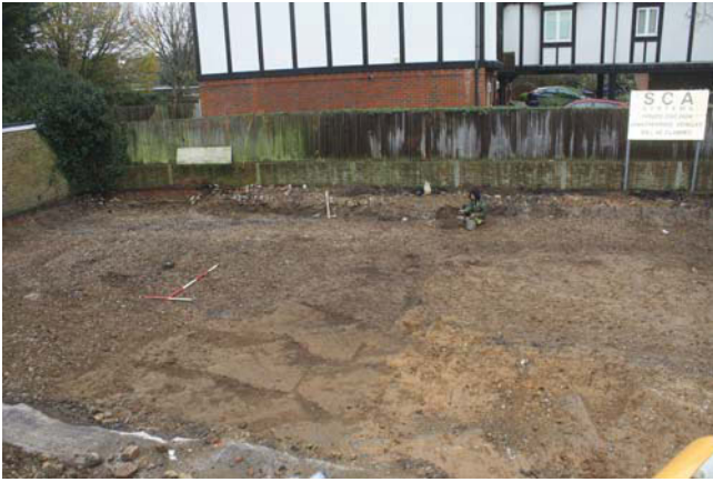
Plate 1. General site view, looking north, Scales: 2m and 1m.
