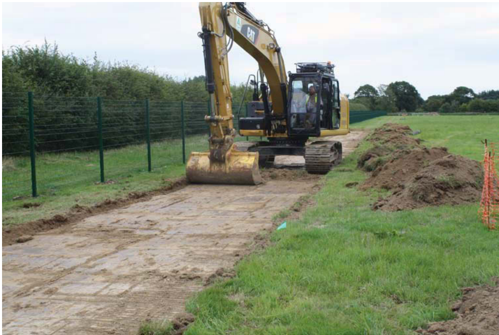
Plate 1. General view of stripping in progress.
