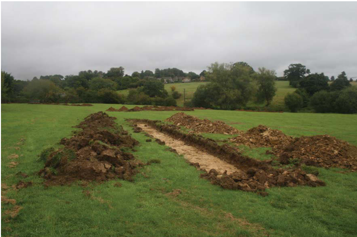
Plate 1. Overview of site, looking east from Trench 7.
