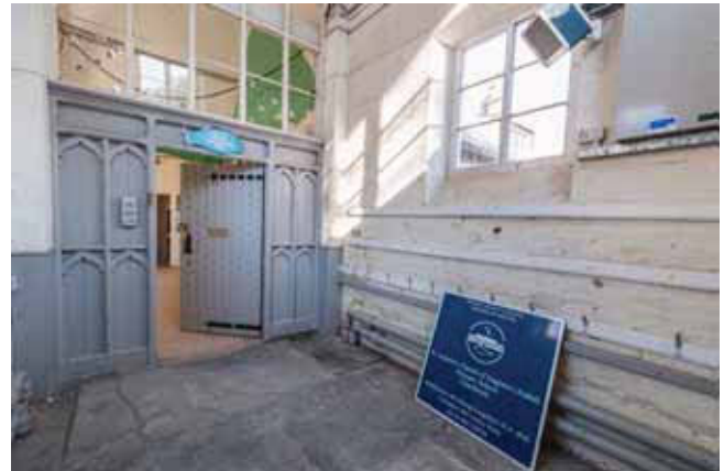
Plate 10. Oblique view of room 4, looking Northeast.
