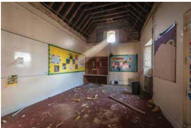
Plate 19. View to window in south gable end, looking South.
