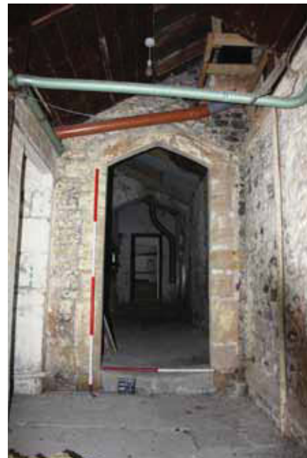
Plate 26. View along corridor, looking East, Scales: 2m and 1m.
