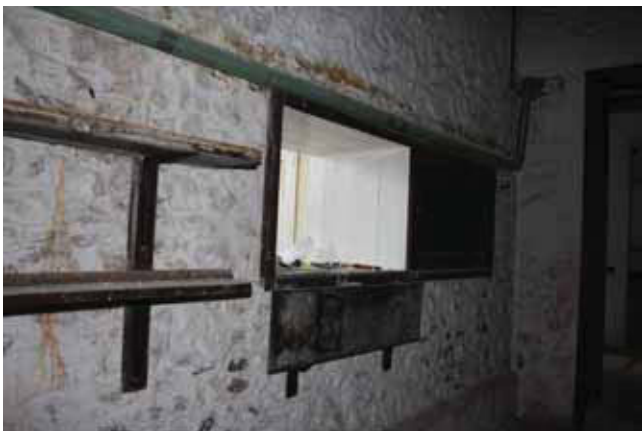
Plate 27. Serving hatch, looking Northeast.
