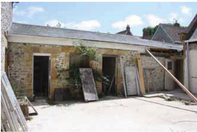
Plate 7. West elevation of east range (within yard area), looking Southeast, Scales: 1m.
