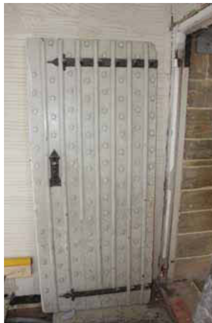
Plate 14. Door detail, looking North.
