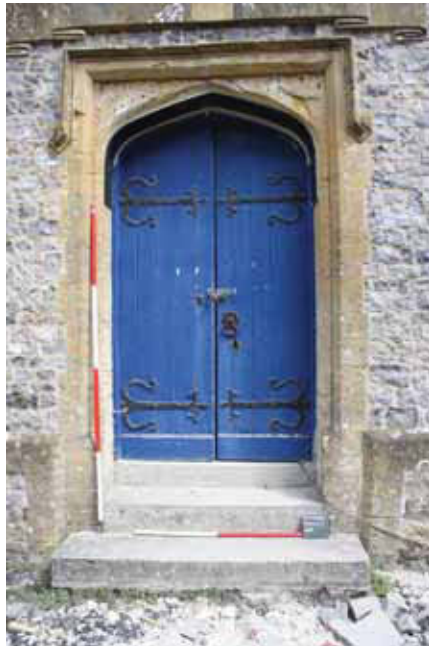
Plate 9. Entrance door to former National School, looking North, Scales: 2m and 1m.
