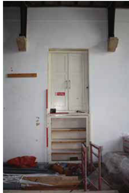
Plate 22. Cupboard within blocked doorway, looking South, Scales: 2m and 1m.
