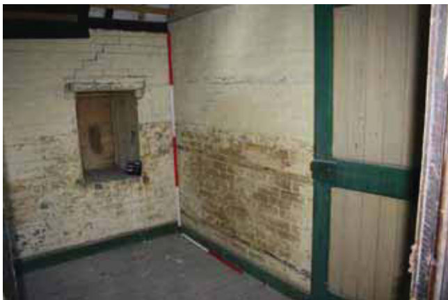
Plate 43. Window in room 25, looking Northwest, Scales: 2m and 1m.
