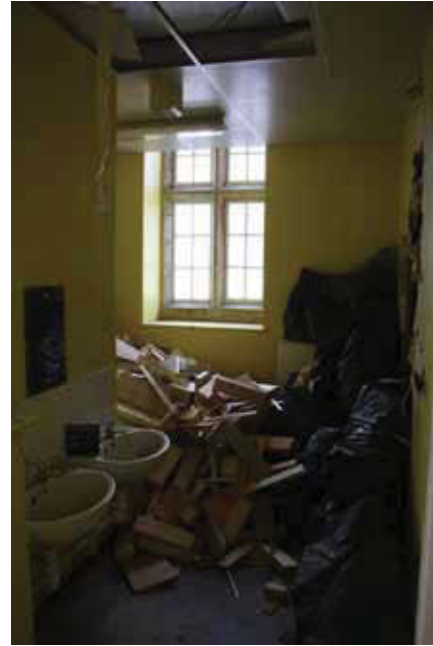
Plate 34. Oblique view to window, looking Northwest.
