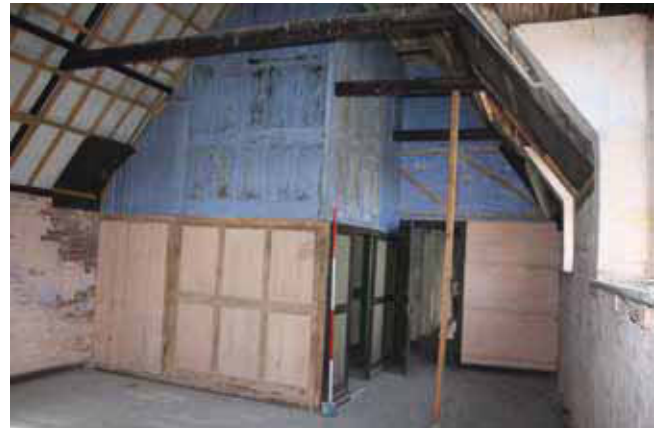
Plate 42. Partition wall detail of room 25, looking Northwest, Scales: 2m and 1m.
