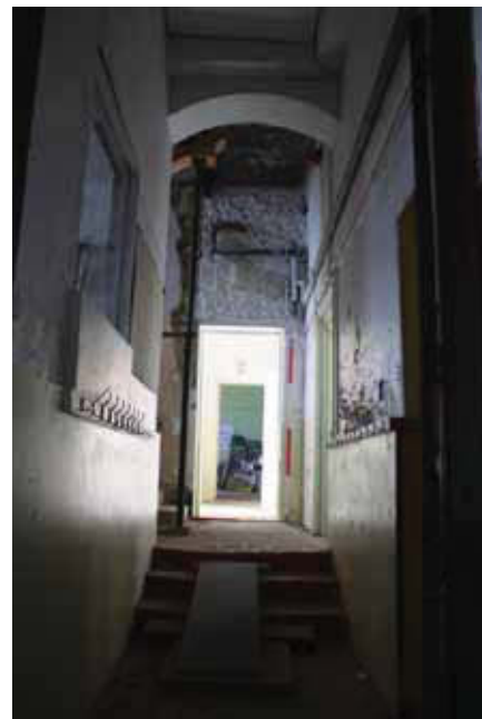
Plate 28. View along corridor, looking East, Scales: 2m and 1m.
