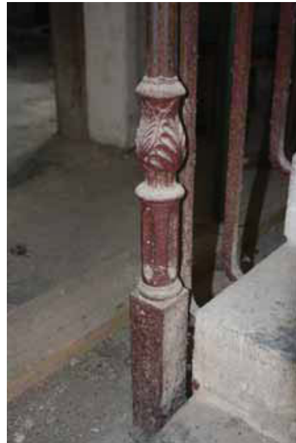
Plate 30. Stair detail, looking North.
