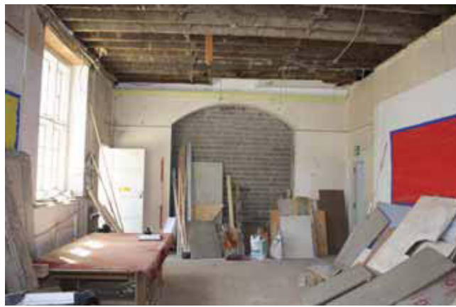
Plate 16. View to blocked arch, looking South, Scales: 2m.
