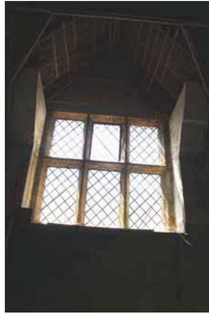
Plate 40. Window detail, looking South.
