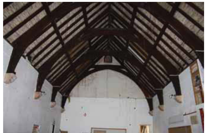
Plate 24. Roof structure, looking East.
