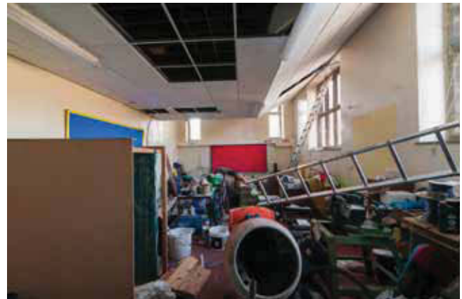
Plate 36. View to windows in west gable end, looking West.
