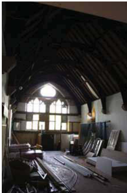
Plate 23. View to west gable end, looking Northwest.
