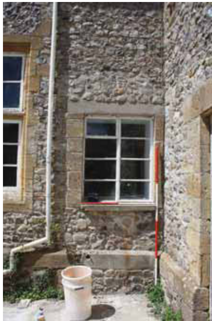
Plate 17. Blocked door (within yard area), looking West, Scales: 2m and 1m.
