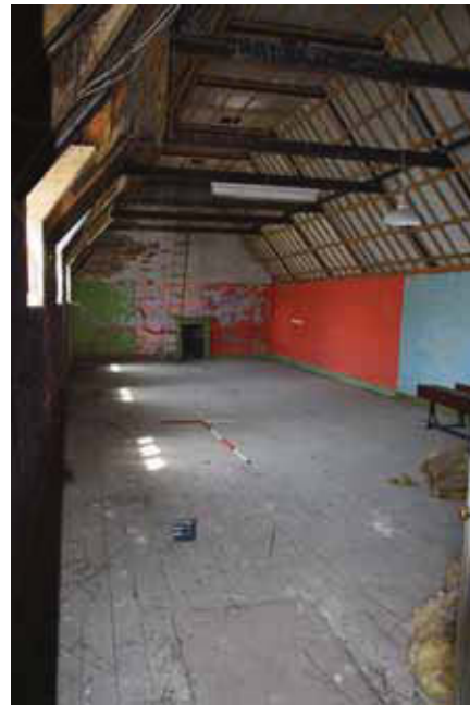
Plate 38. General view of room, looking Northwest, Scales: 2m and 1m.
