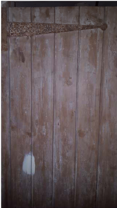
Plate 15. Detail of door with strap hinge looking Southeast.
