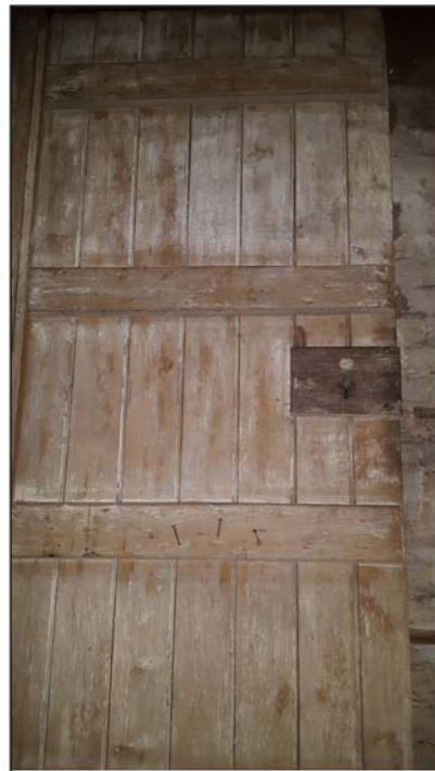
Plate 16. Detail of door with strap hinge looking Southeast.
