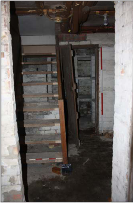
Plate 13. View to stairs and shelving, looking Northeast, Scales: 2m and 0.5m.
