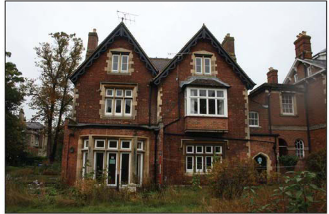
Plate 6. Rear elevation, looking Northwest, Scale: 2m.
