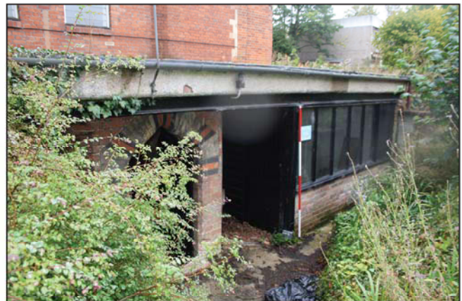
Plate 4. Cellar oblique, looking East, Scale: 2m.
