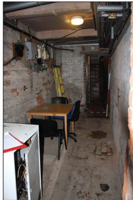
Plate 8. General view of room 2, looking Northeast, Scales: 2m and 0.5m.
