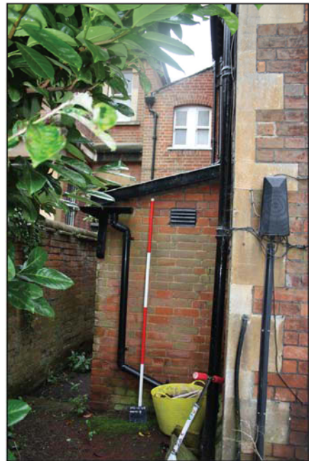
Plate 2. Front elevation, east side, looking Southeast, Scale: 2m.
