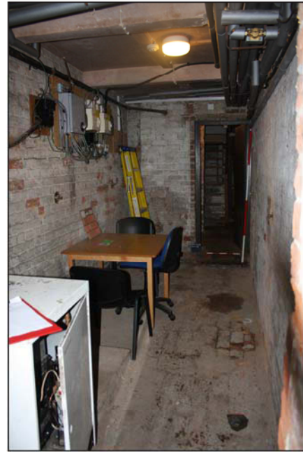
Plate 10. General view of room 2, looking Northeast, Scales: 2m and 0.5m.
