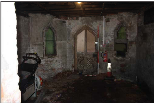
Plate 7. View to bay window/entrance, looking Southwest, Scales: 2m and 0.5m.
