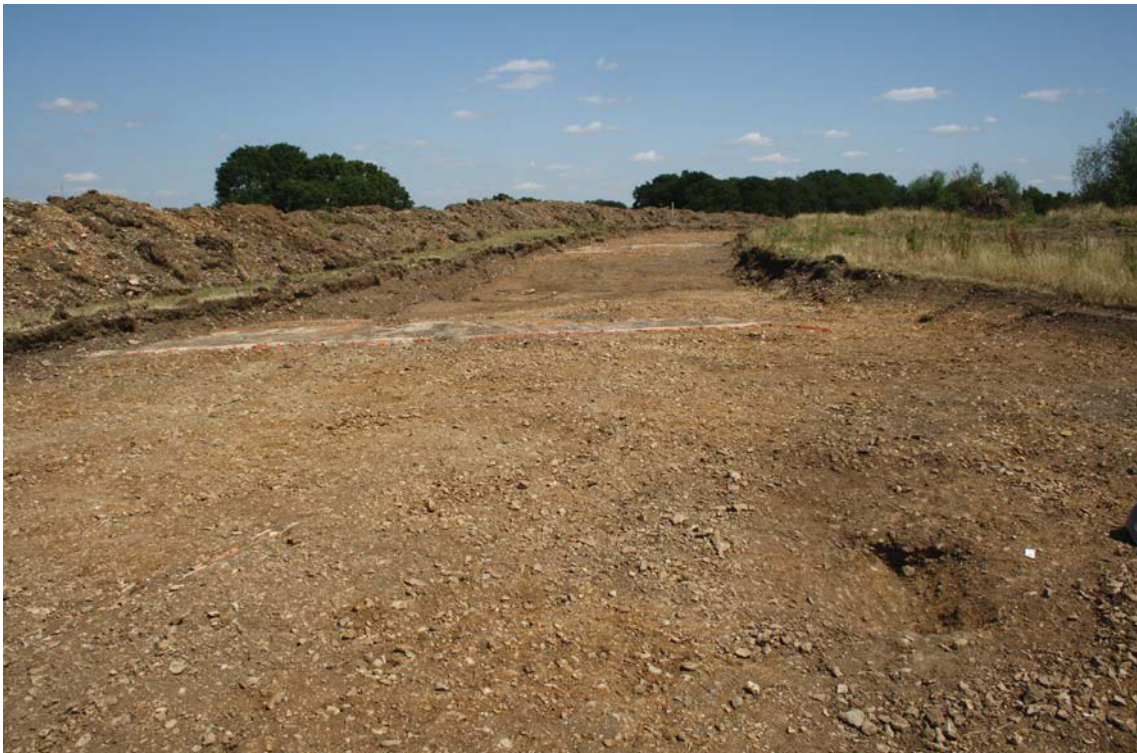
Plate 1. Site looking uphill from structure 452, looking east.
