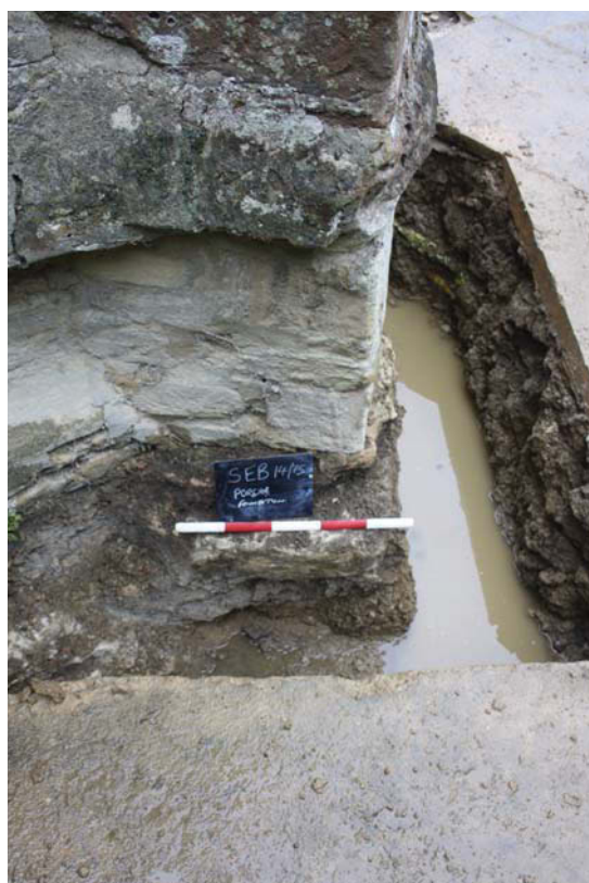
Plate 2. North east buttress foundation on porch, looking west, Scale: 0.5m.
