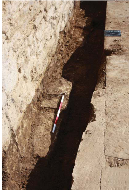
Plate 7. Foundation on South Aisle Chapel, Scale: 0.5m.
