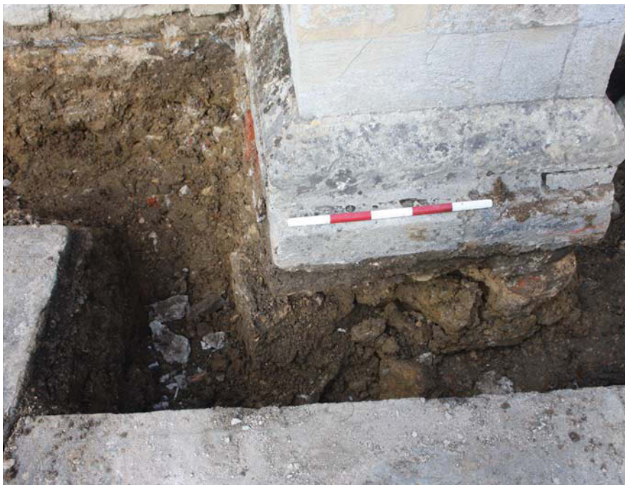
Plate 8. South Aisle buttress foundation , Scale: 0.5m.
