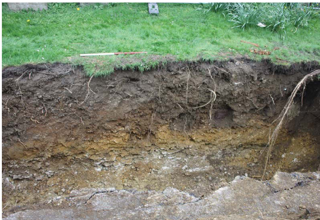
Plate 1. Soakaway section, looking west, Scale: 1m.
