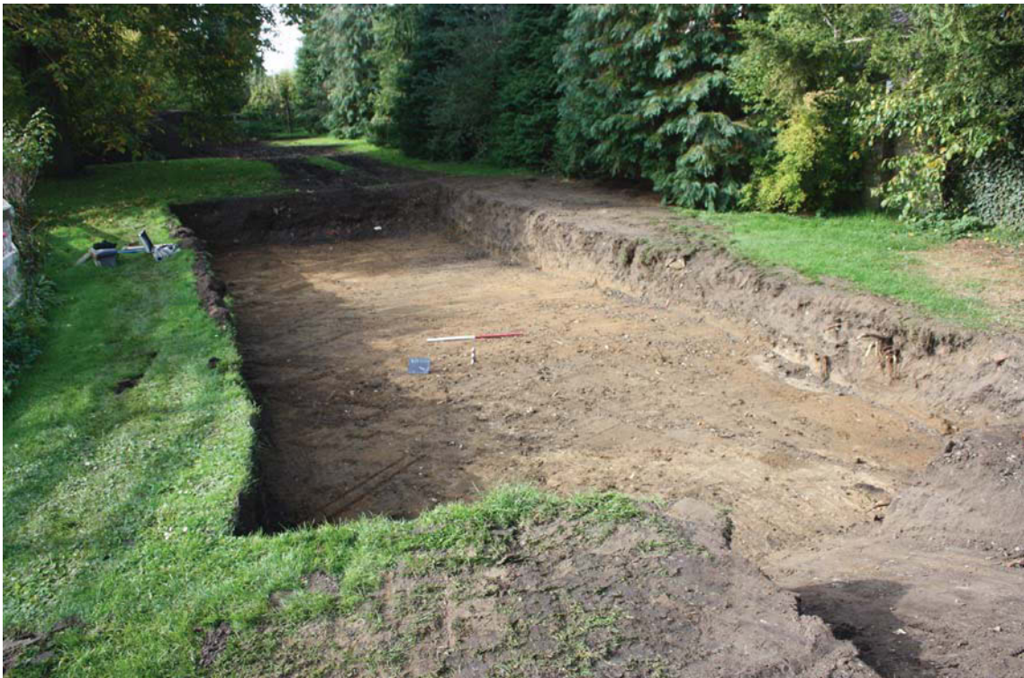
Plate 1. House strip, looking south west, Scales: 1m and 0.5m.
