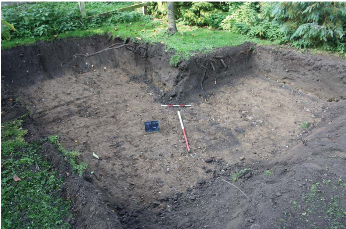
Plate 2. Garage strip, looking west, Scales: 1m and 0.5m.
