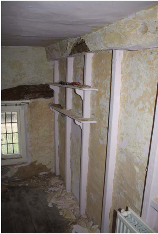
Plate 9. Bedroom C during building work, looking S.
