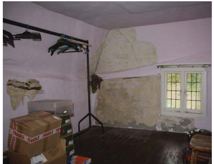
Plate 4. Bedroom C, looking SSE.
