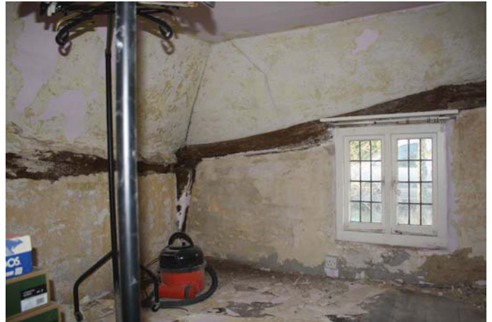
Plate 8. Bedroom C during building work, looking SSE.
