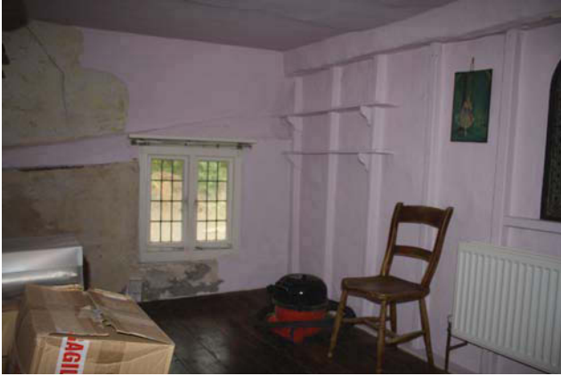
Plate 5. Bedroom C, looking SW.
