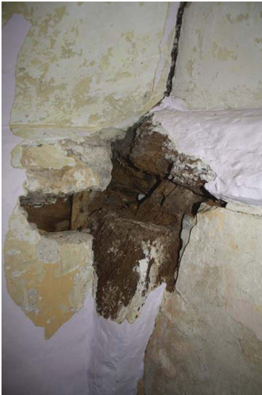
Plate 7. Bedroom C, detail of timber framing in SE corner, looking E.
