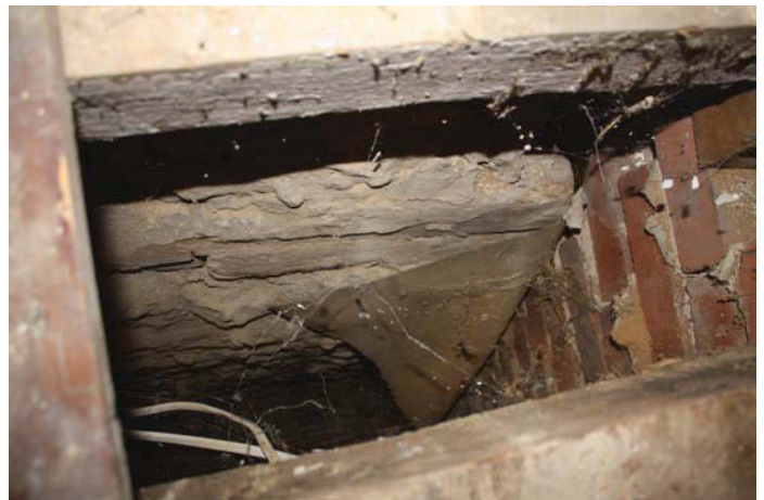
Plate 12. Bedroom C during building work, void below floorboards in SW corner.
