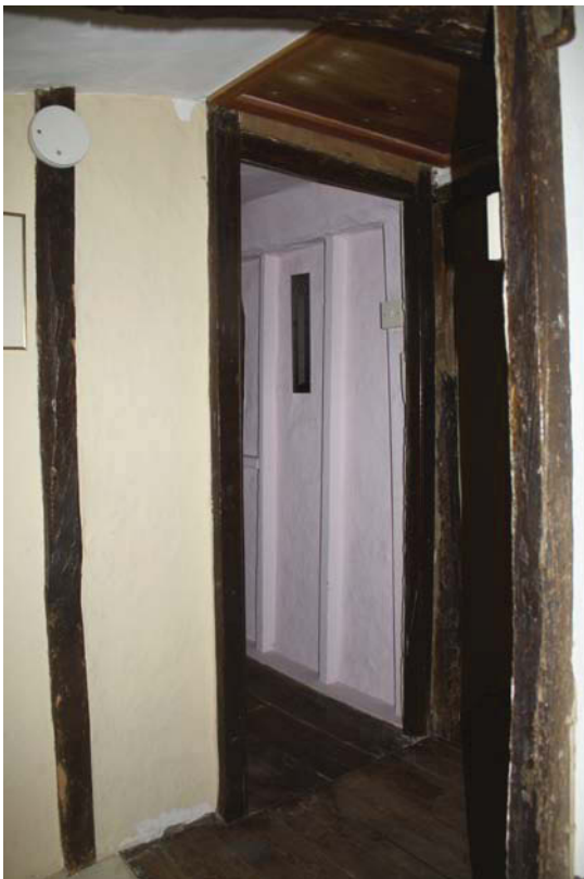
Plate 3. First floor, looking SSW towards bedroom C.
