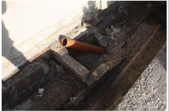
Plate 2. Drain 51 and silt trap 52
