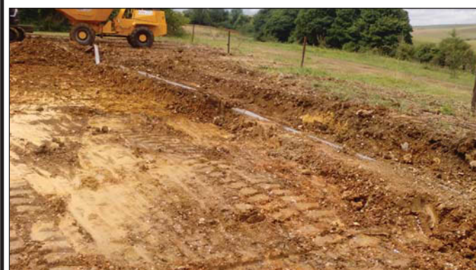
Plate 5: Stripped area, looking north-west.
