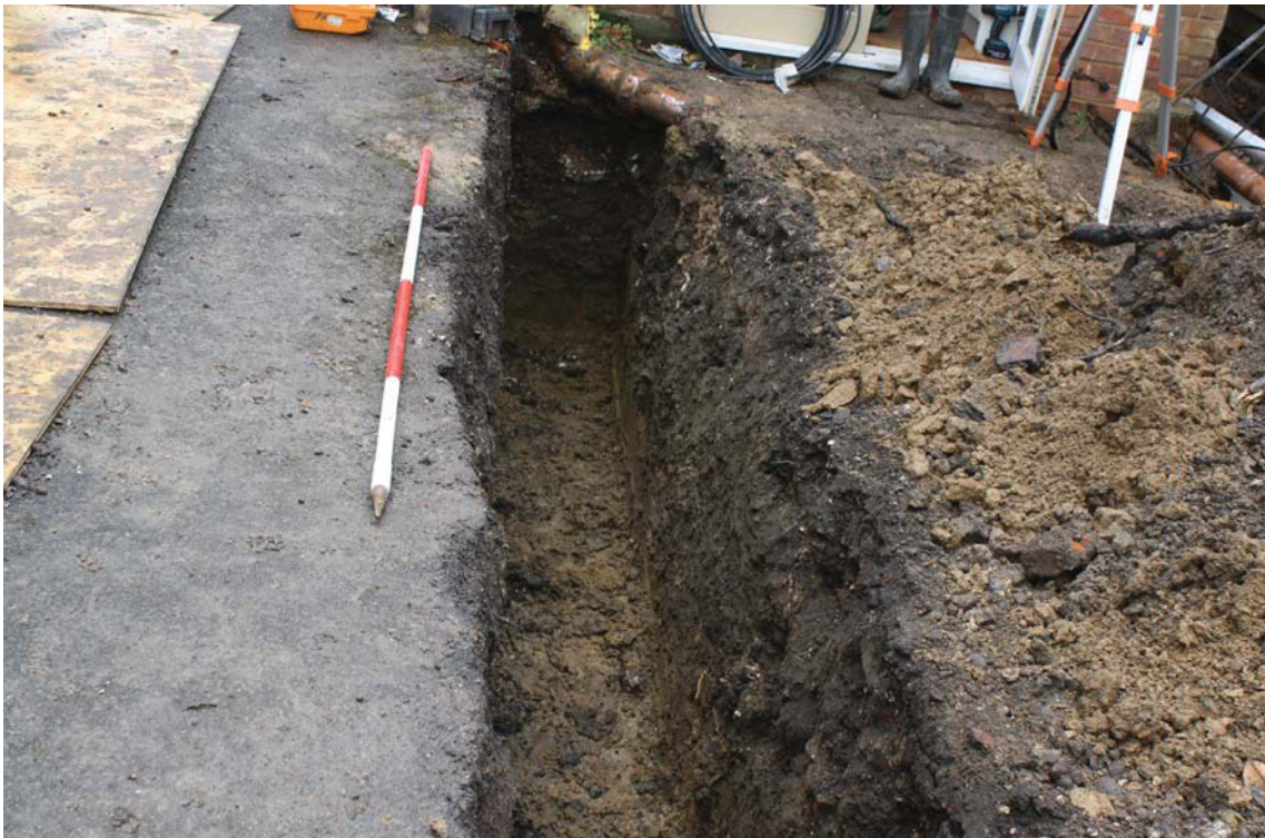
Plate 1. Full excavated depth of footing, looking south, Scale: 2m.
