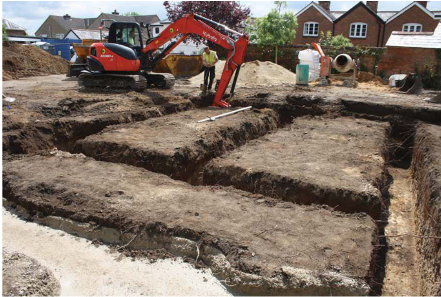
Plate 3. footings, looking south.
