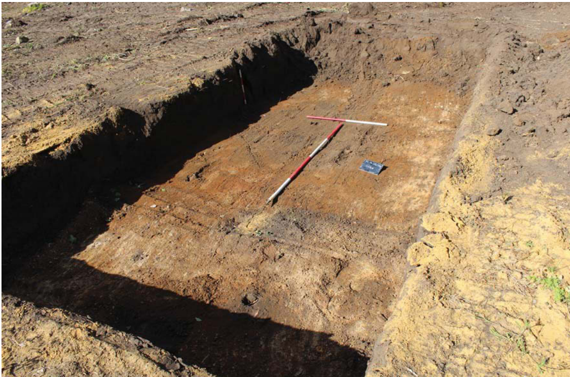
Plate 1. Soakaway 1, looking southeast, Scales: 2m, 1m and 0.5m.
