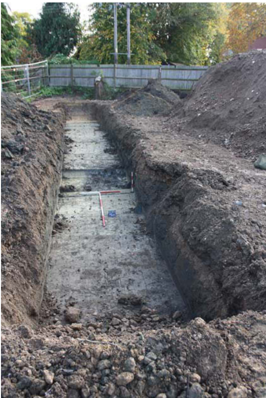
Plate 4. Trench 7, looking east, Scales: horizontal 2m and 1m, vertical 0.5m.
