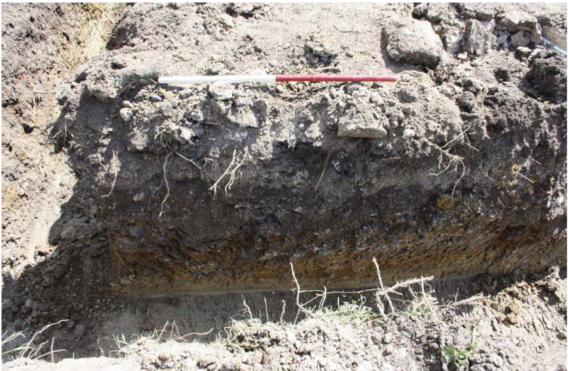
Plate 4. Deep 1.8m footings, looking south west.
