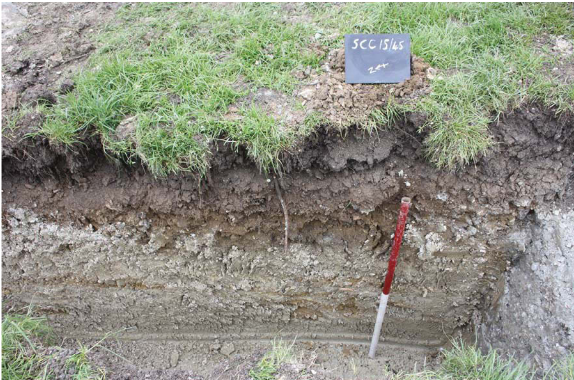
Plate 3. Representative of 1.2m deep footing, looking south east, Scale: 1m.
