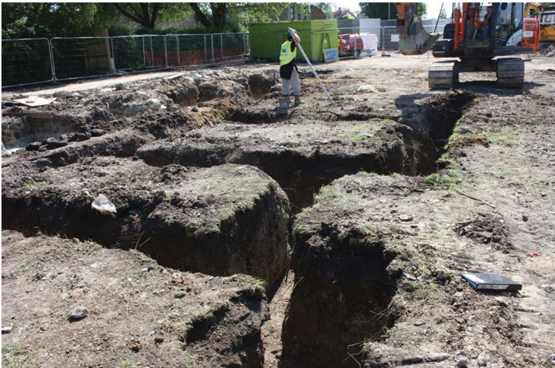
Plate 2. Deep 1.8m footings, looking west.
