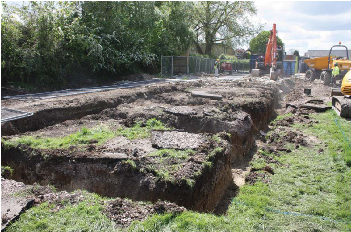
Plate 1. General shot over footings, looking west.
