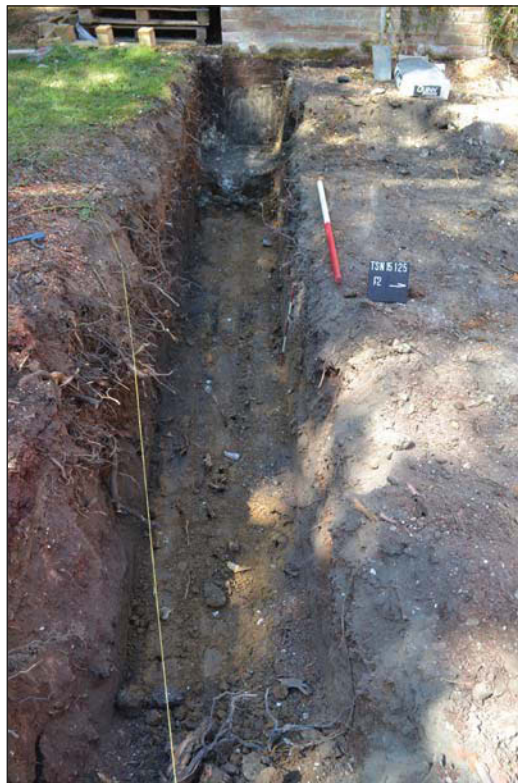
Plate 2. Southern footing trench looking west, Scales: 1m and 0.5m.
