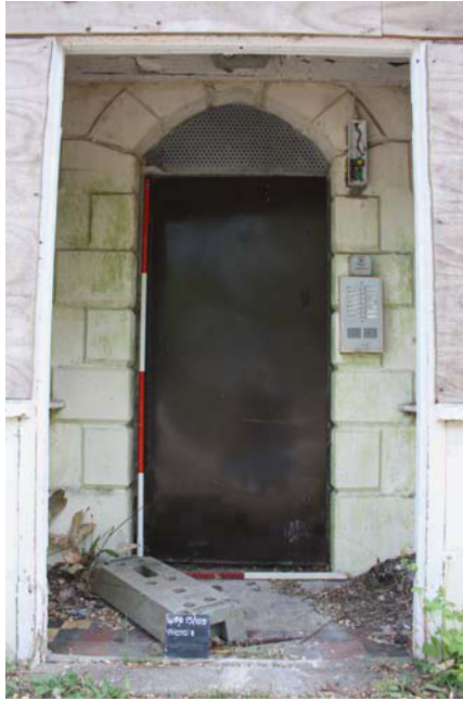
Plate 11. Door detail, looking East, Scales: 2m and 1m.
