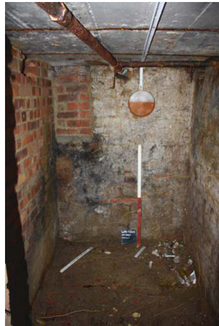
Plate 16. Stone walling detail, looking East, Scales: 2m and 1m.
