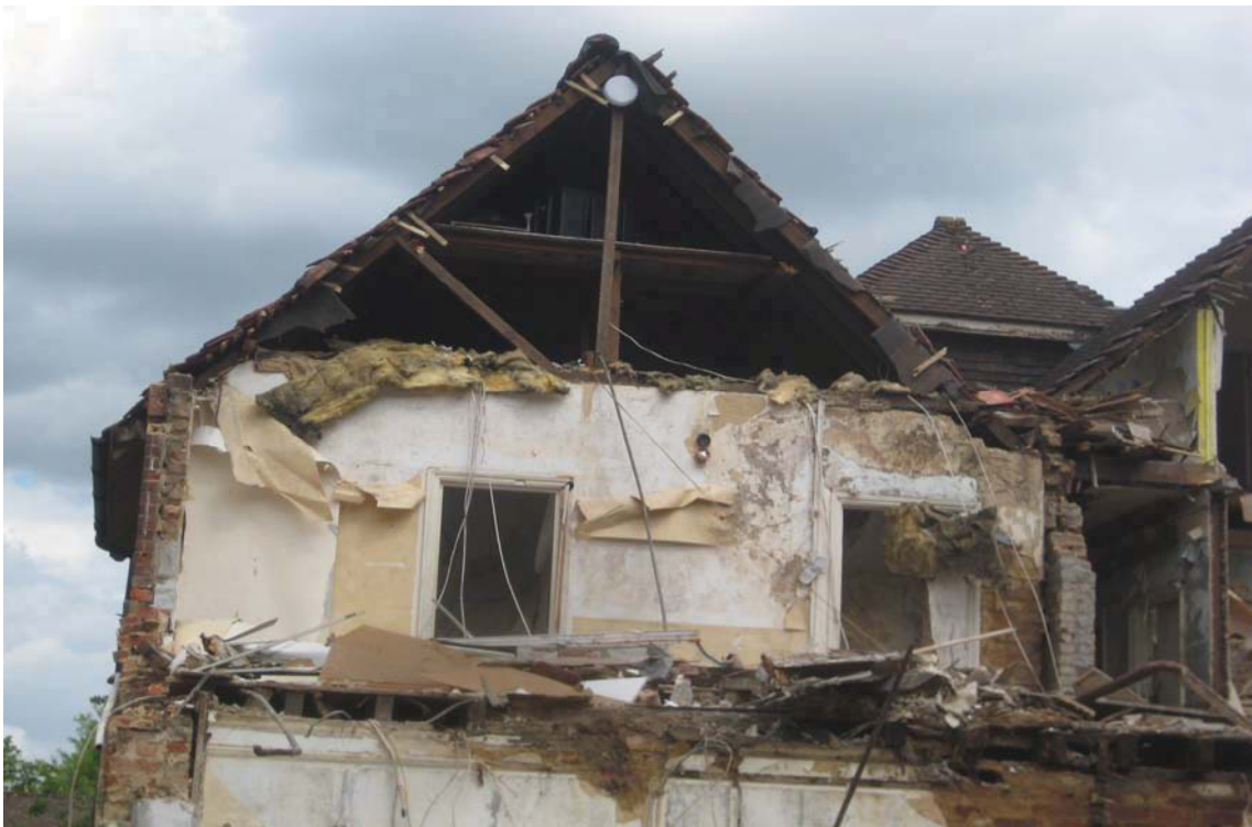
Plate 32. North gable roof structure, looking East.
