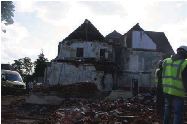
Plate 29. Partial demolition of north gable rooms (Rms 6 and 18), looking East.
