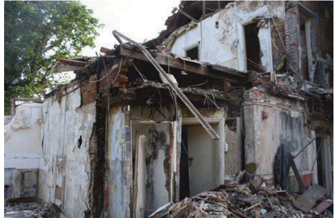
Plate 20. False ceiling and blocked doorway, looking Northeast.
