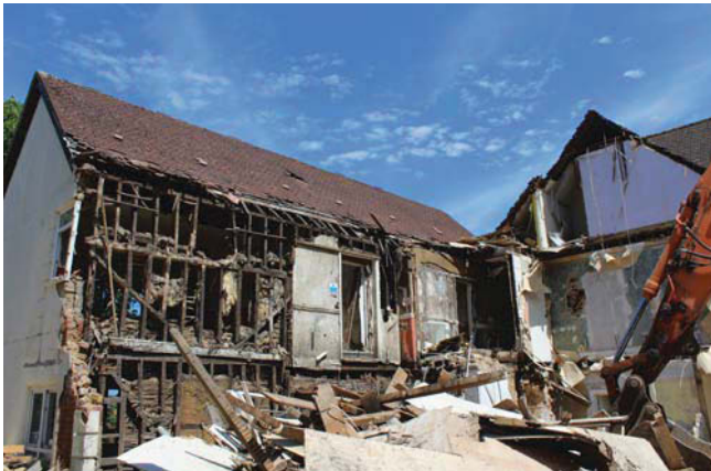
Plate 17. Detail of timber framing in N. gable (Rm 17), looking Northeast.
