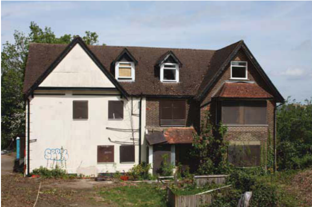
Plate 7. South elevation, looking North, Scales: 2m and 1m.
