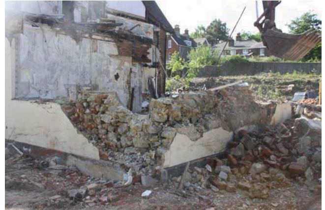
Plate 4. Rubble and brick wall in the NW gable end (Rm 6) looking southeast.
