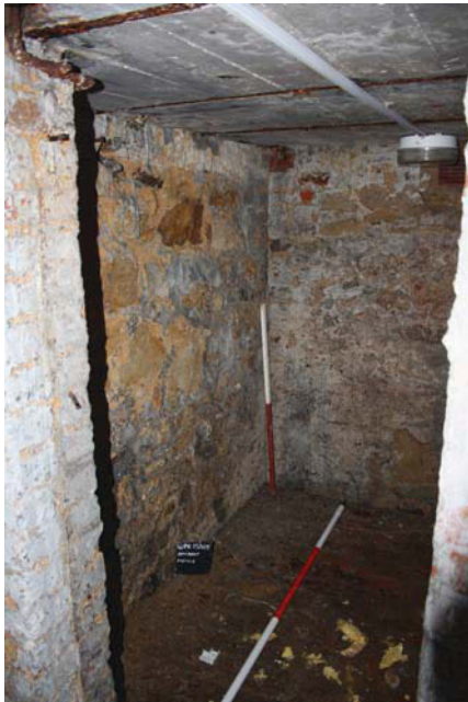
Plate 15. Stone walling detail, looking East, Scales: 2m and 1m.
