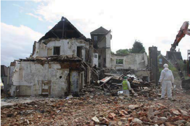
Plate 27. View of first floor (Rms 8 and 16), looking East.
