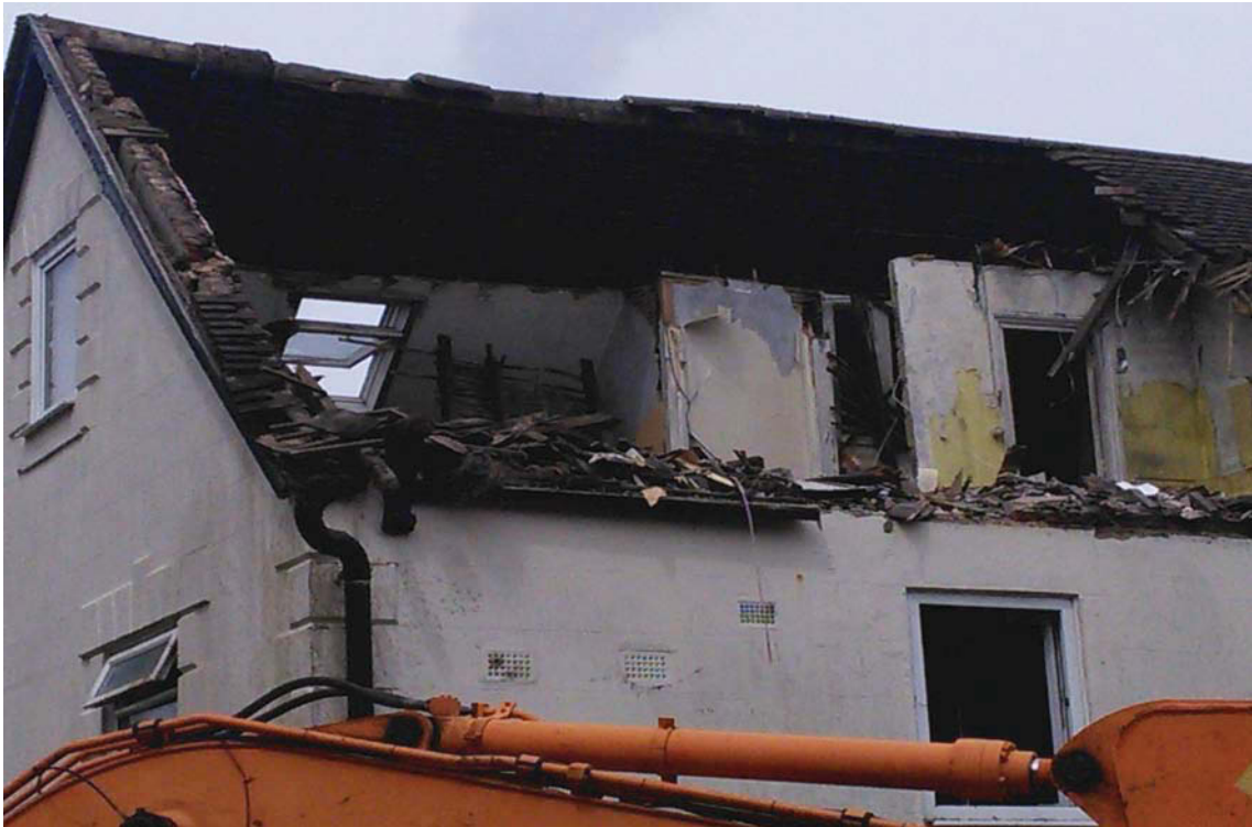
Plate 31. Roof construction (Rm 21), looking Northeast.
