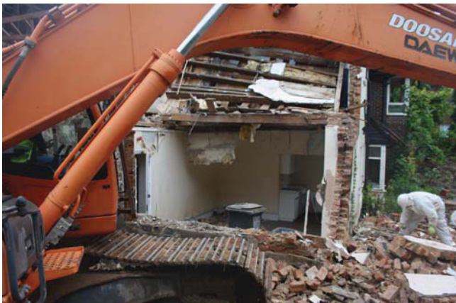
Plate 21. Detail of ground floor rooms in S. gable (Rm 7), looking East.
