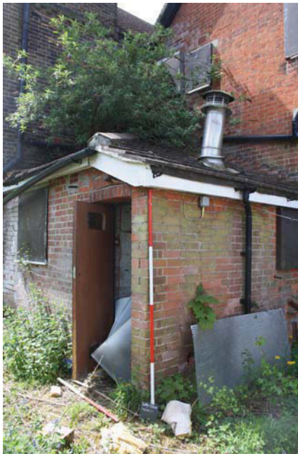
Plate 5. Oblique of west elevation, looking Southwest, Scales: 2m and 1m.
