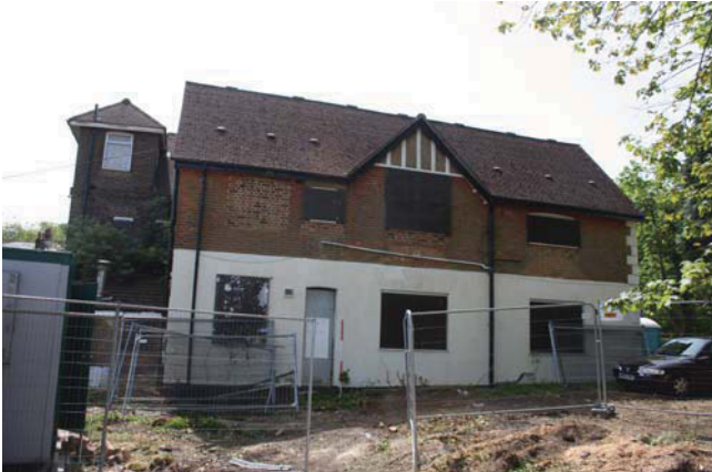
Plate 3. North elevation, looking South, Scales: 2m and 1m.
