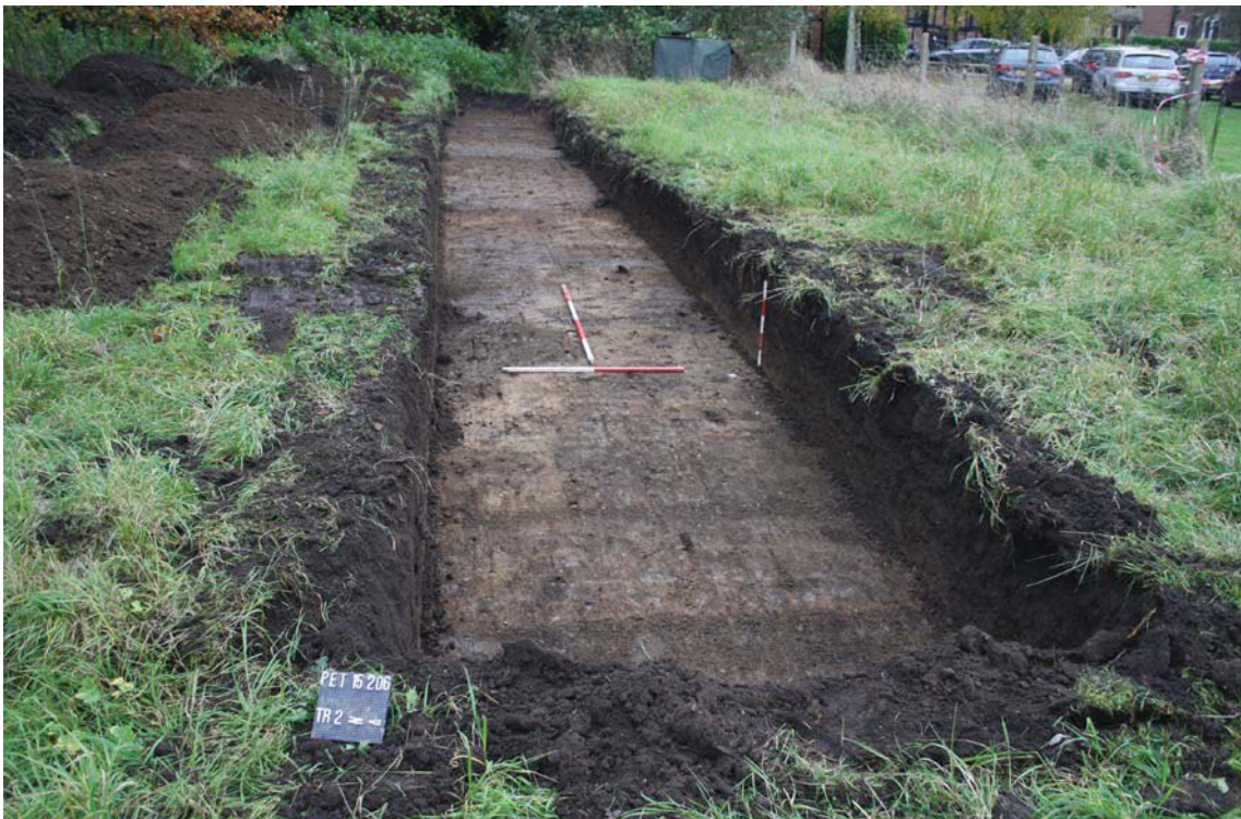
Plate 2. Trench 2, looking east south east, Scales: horizontal 2m and 1m, vertical 0.5m.
