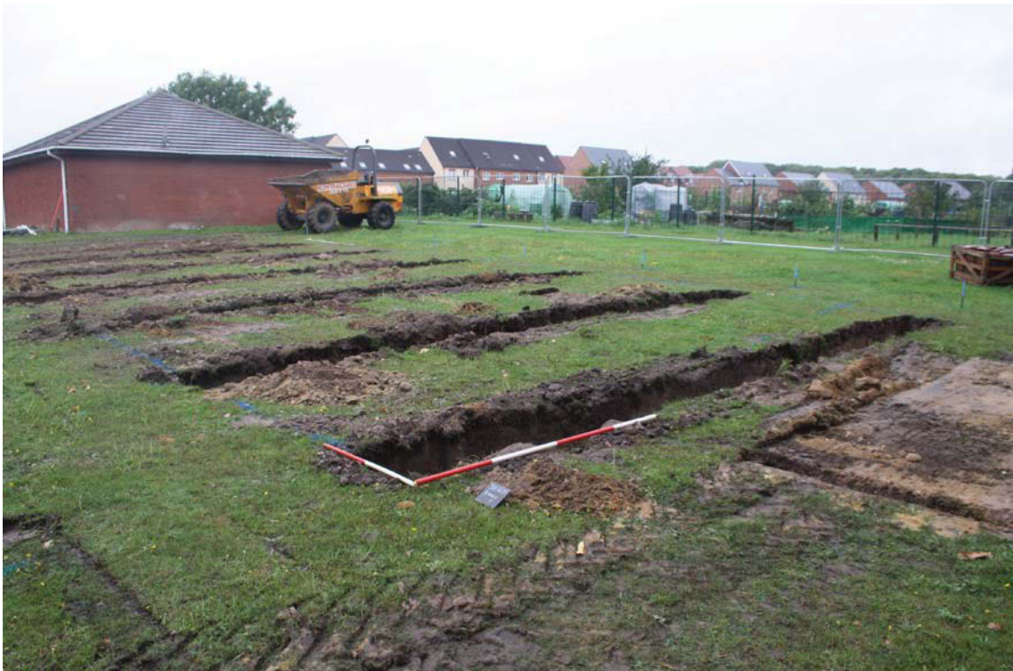
Plate 1. View over building foundation trenches, looking west, Scales: 2m and 1m.
