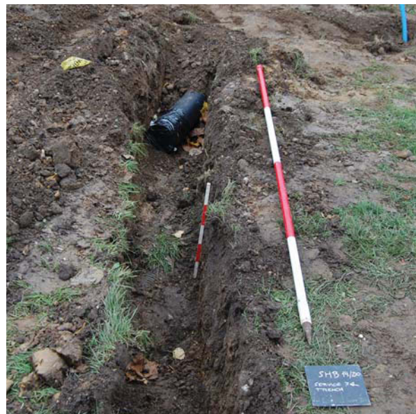
Plate 3. Service trench, looking east, Scales: 2m and 0.5m.
