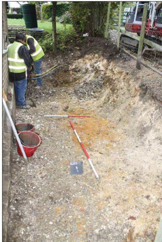
Plate 2. Exterior ground reduction in east, looking north, Scales: 2m and 1m.
