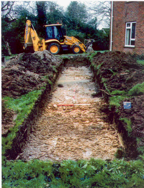
Plate 2. Trench 3, looking north west, Scales 1m and 2m.
