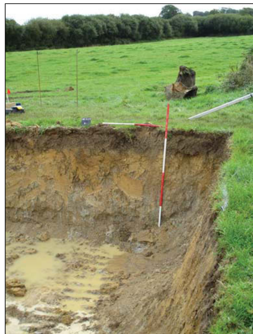
Plate 4. DPV substation base section looking east, Scales: 2m and 1m.
