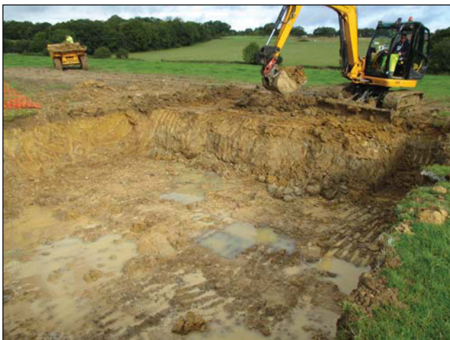
Plate 3. DPV substation base during final stages of excavation, looking north west
