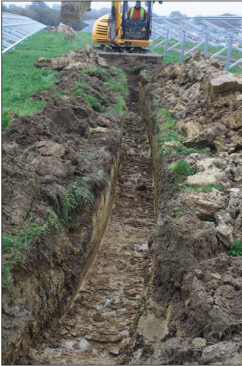
Plate 1. Cable trench in Area B looking east during excavation
