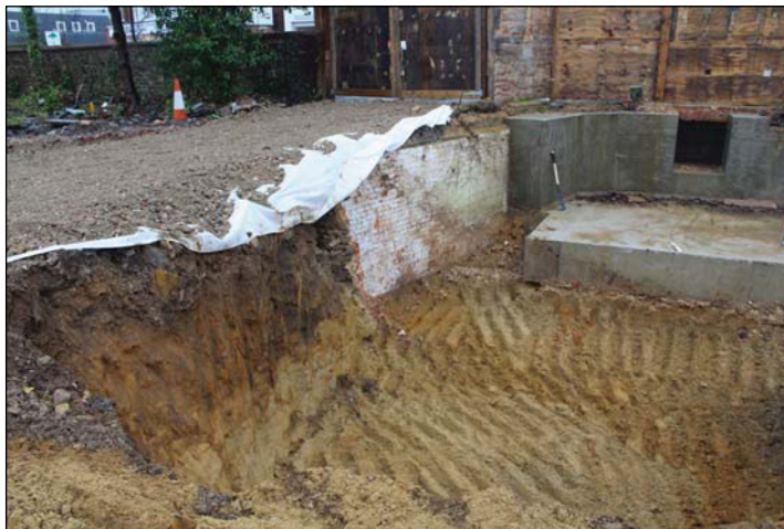
Plate 3. Area of former basement looking north east
