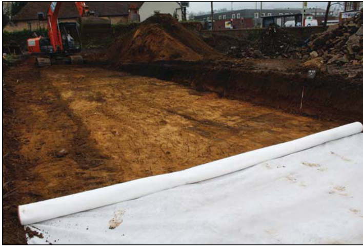
Plate 1. View of part of stripped area looking north west, Scale: 0.5m
