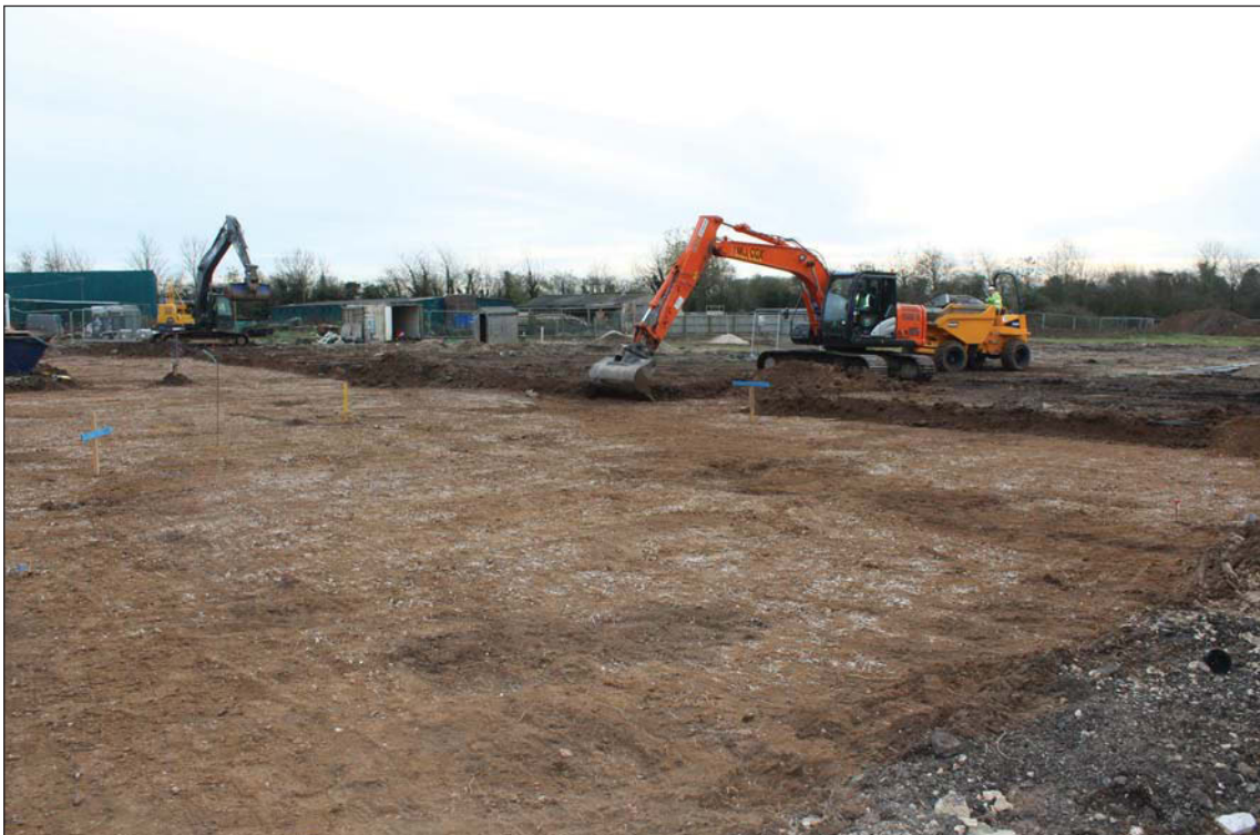
Plate 2. Overburden stripping revealing ditch looking south west.
