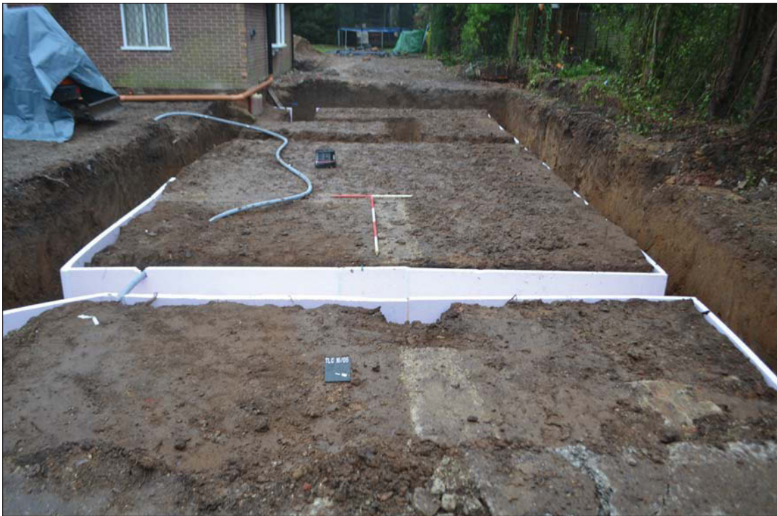
Plate 3. Foundations, looking south-west, Scales: 2m and 1m.
