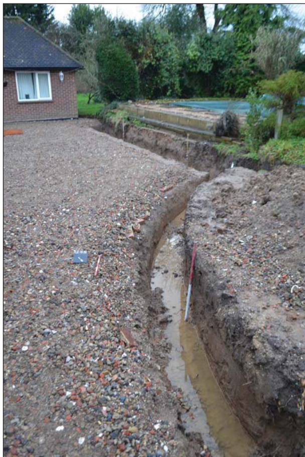
Plate 1. Retaining wall trench, looking south-west, Scales: 1m and 0.5m.
