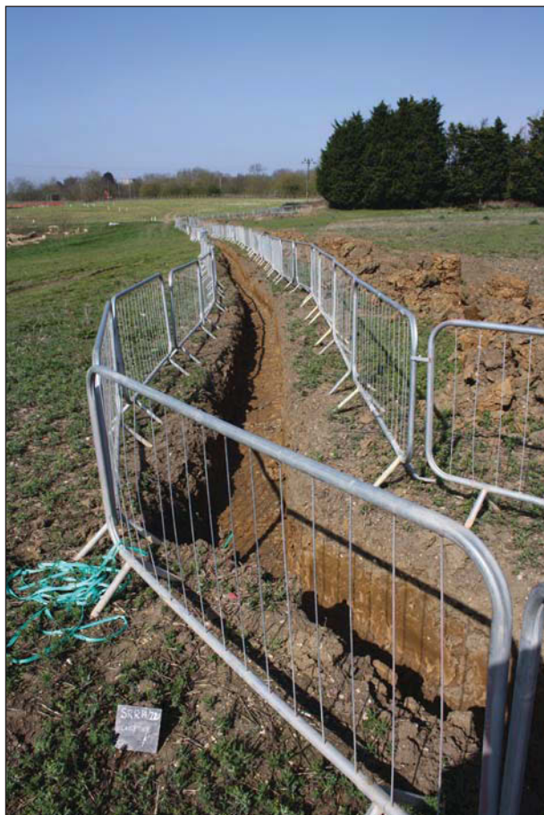
Plate 5. Cable Trench, looking north west.
