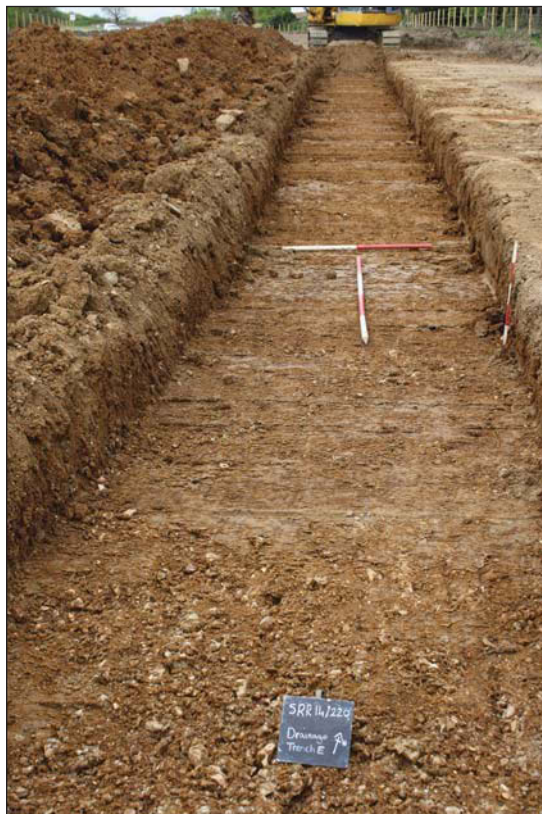
Plate 8. Eastern Road Trench, looking north-northwest, Scales: 2m, 1m and 0.5m.
