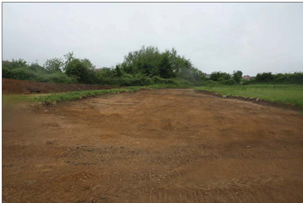
Plate 10. General view of road strip spur, Area C looking east.
