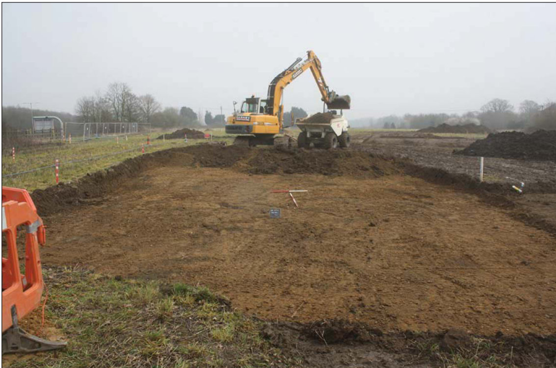
Plate 3. Gas main strip, looking north east, Scales: 2m and 1m.
