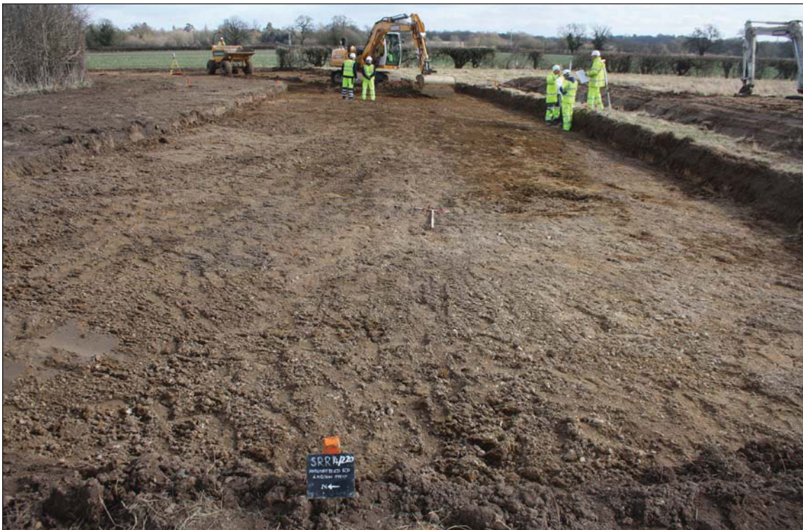
Plate 2. Lagoon area strip, looking north.
